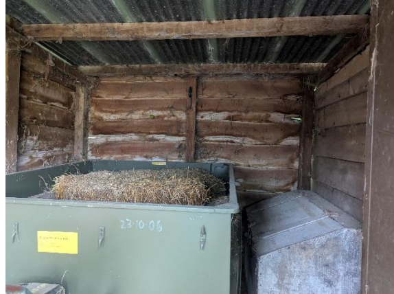
Photo 2 – internal view of field shelter, southern side
