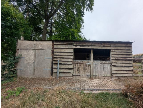
Photo 1 – external view of the field shelter, east elevation
