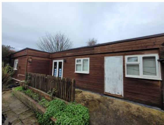
Photo 2: The southern elevation of the surveyed building.
