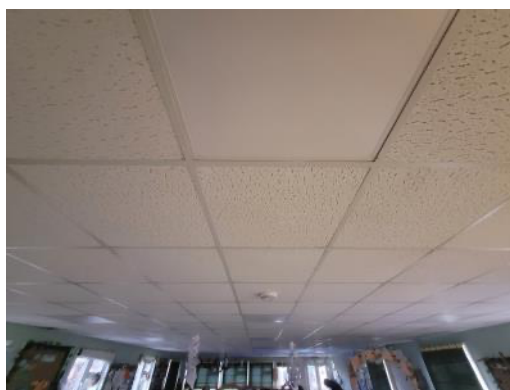
Photo 4: An internal view of the surveyed buildings suspended ceiling.
