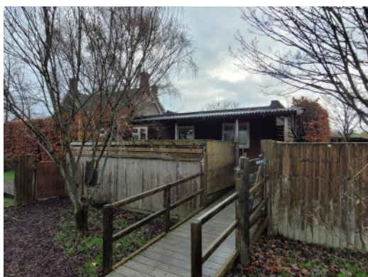
Photo 3: The surveyed building and rear decking viewed from the north-west.
