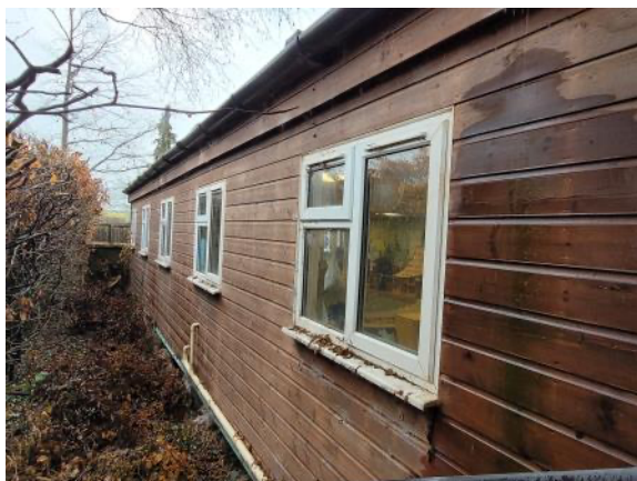
Photo 1: The northern elevation of the surveyed building.
