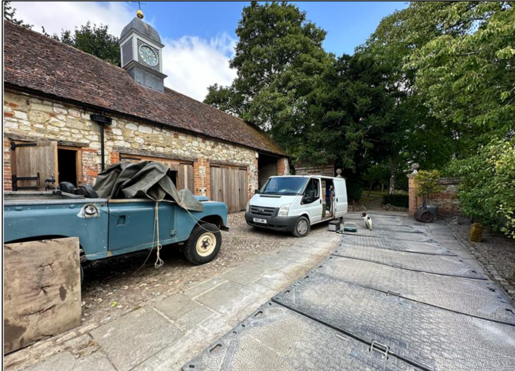
Fig.5 –Grade II listed Stables currently providing supplementary storage and parking
