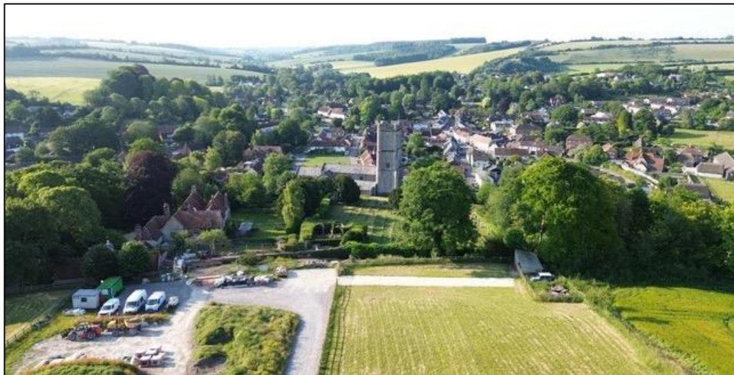
Fig.7 – Application site as existing. The gravelled areas currently form part of a temporary builders' compound associated with the ongoing construction of the swimming pool within the grounds of The Court House.
