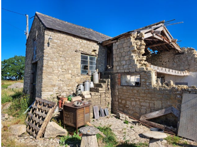
Photo 6 – View of the front/side elevation (east)
