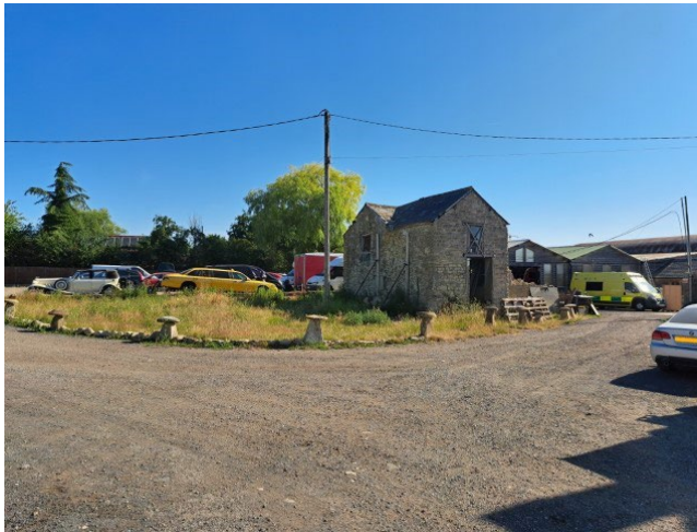
Photo 4 – View of the front/side elevation of the barn (southwest)
