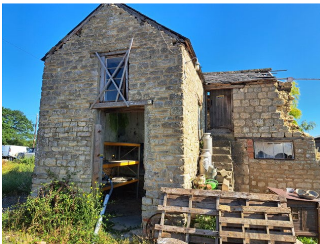
Photo 5 – View of the front elevation (south)
