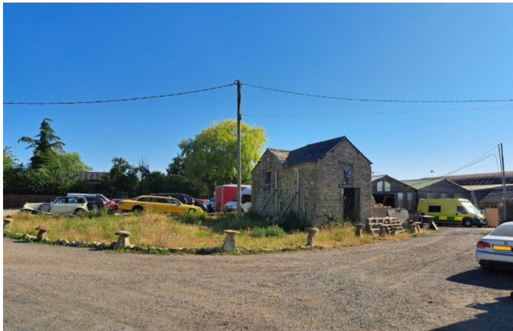
Photo 1 – View of the front/side elevation of the dairy barn
