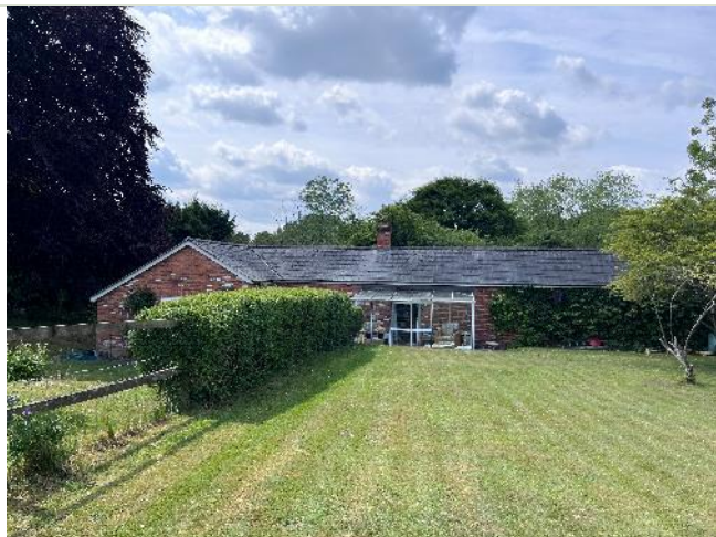
The surveyed bungalow and workshop
