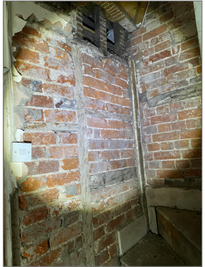
Image 28: Stairwell at Ground Floor
