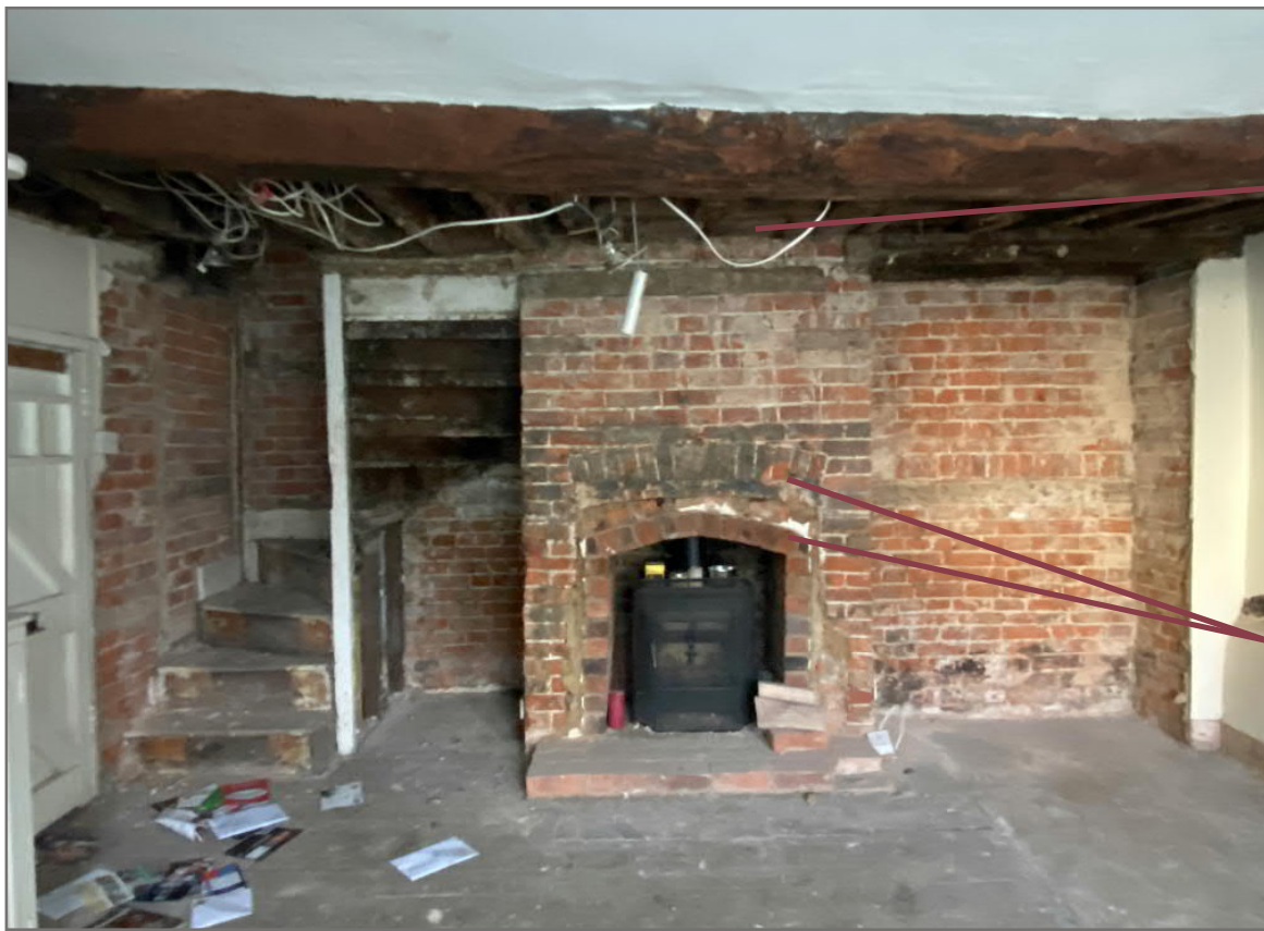
Image 17: View of ground floor room, facing east
