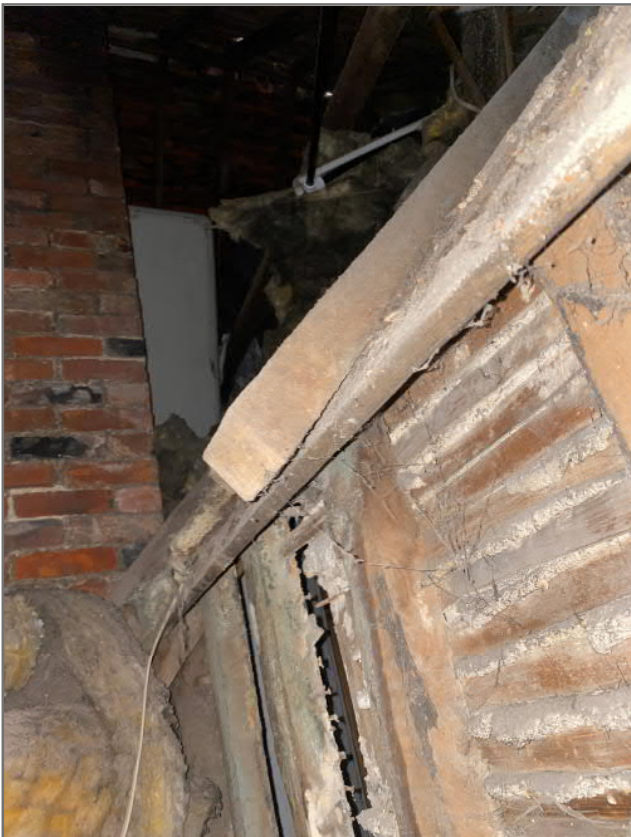
Image 43: View south behind under-eaves cupboard and adjacent chimney breast
