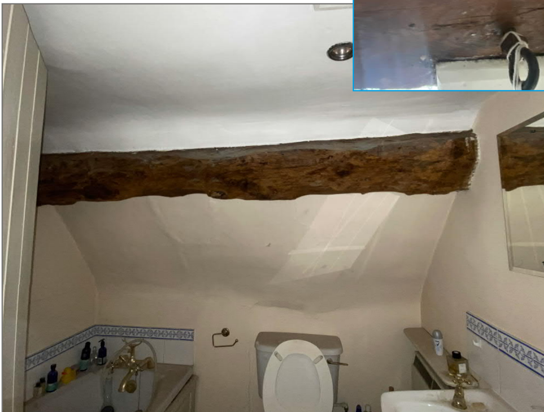
Image 40: View west of purlin in bathroom
