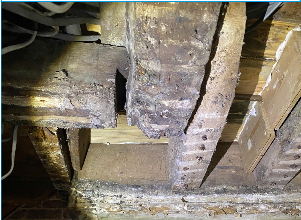
Image 22b: Detail view of underside of staircase
