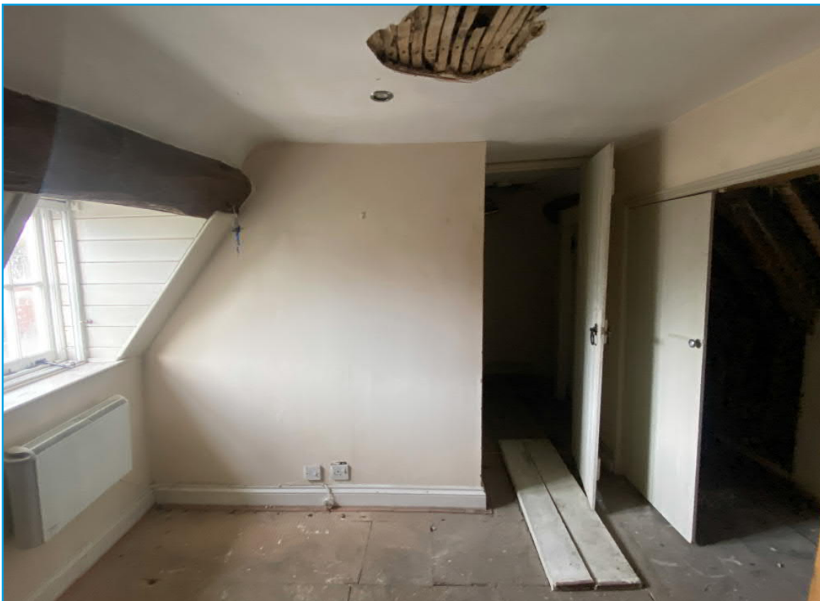
Image 38: View north at Attic Floor
