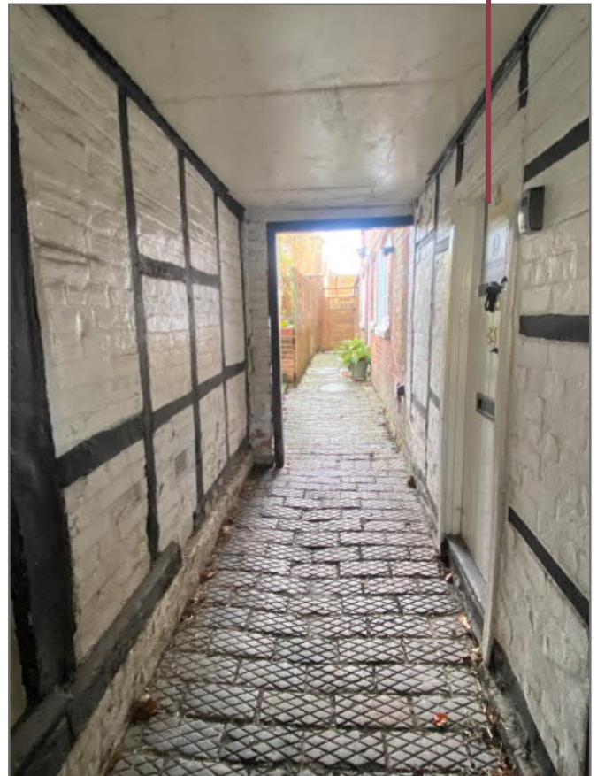
Image 16: View of along passage way towards rear of plot
