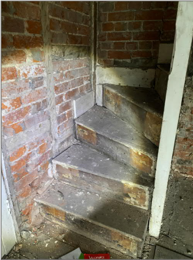
Image 27: Staircase at Ground Floor
