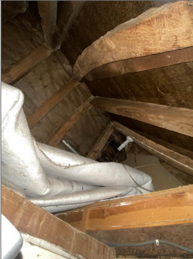
Image 41: View into roof space - common rafters with bridled joints (no ridge beam)
