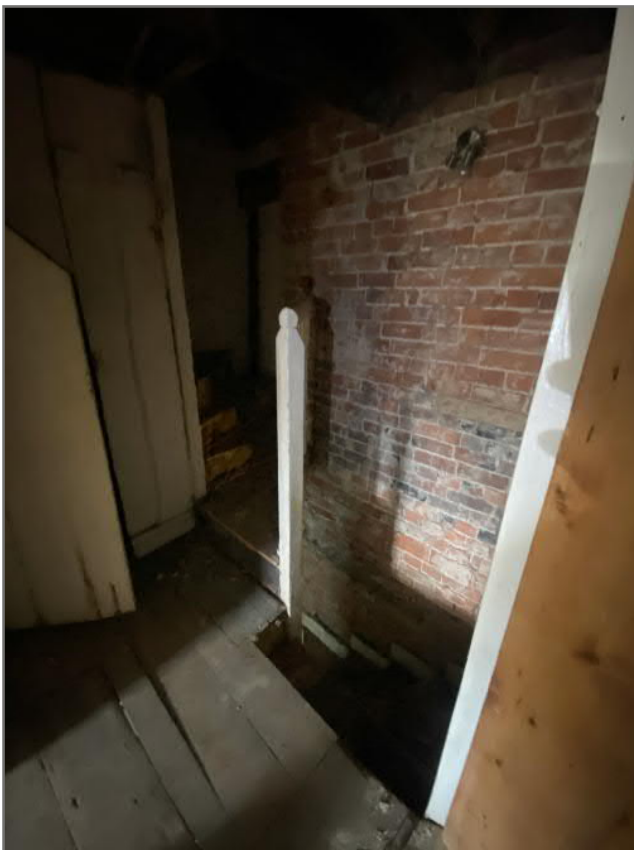
Image 29: View at First Floor of staircase/well
