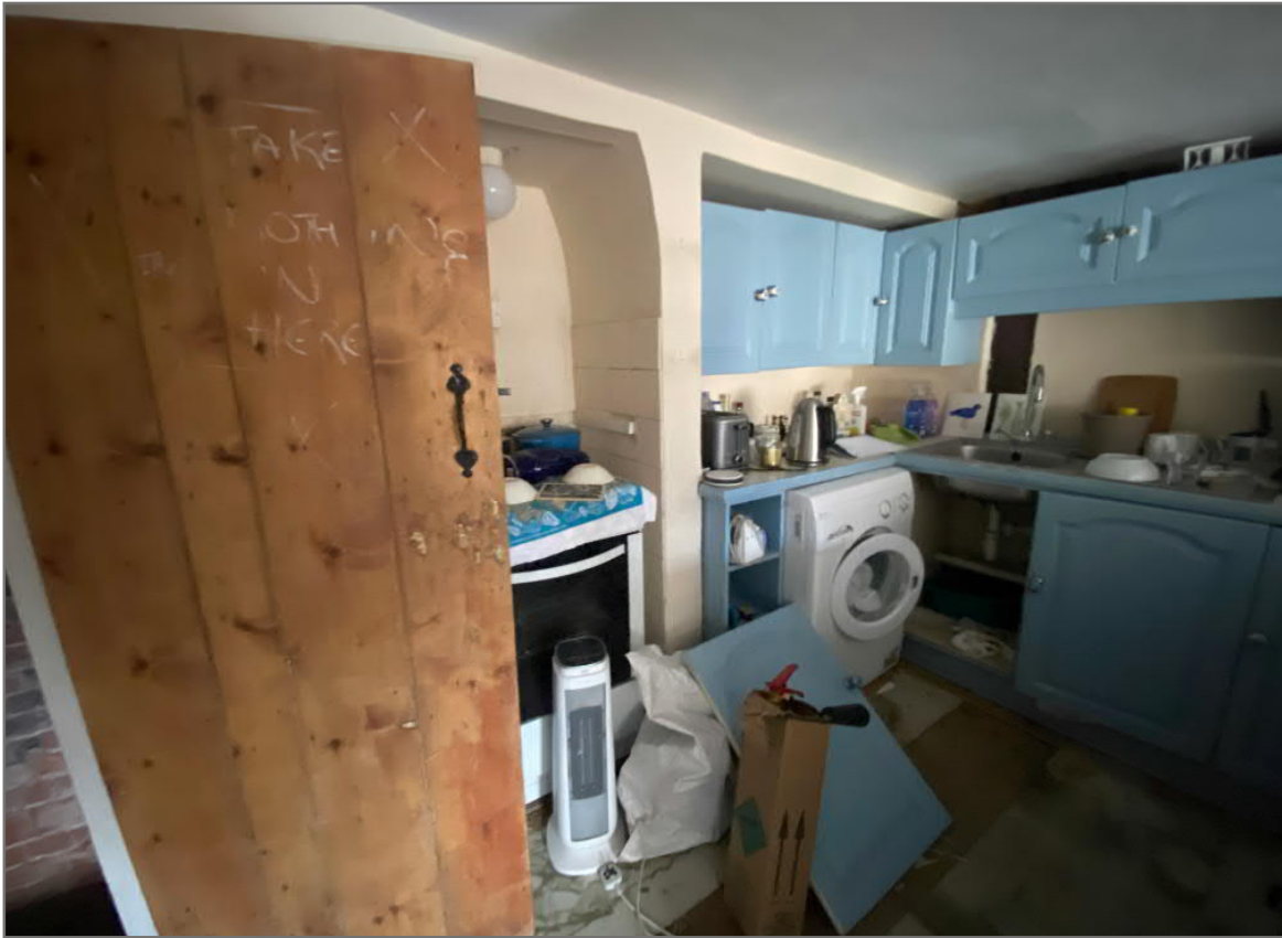
Image 31: View of south wall at First Floor
