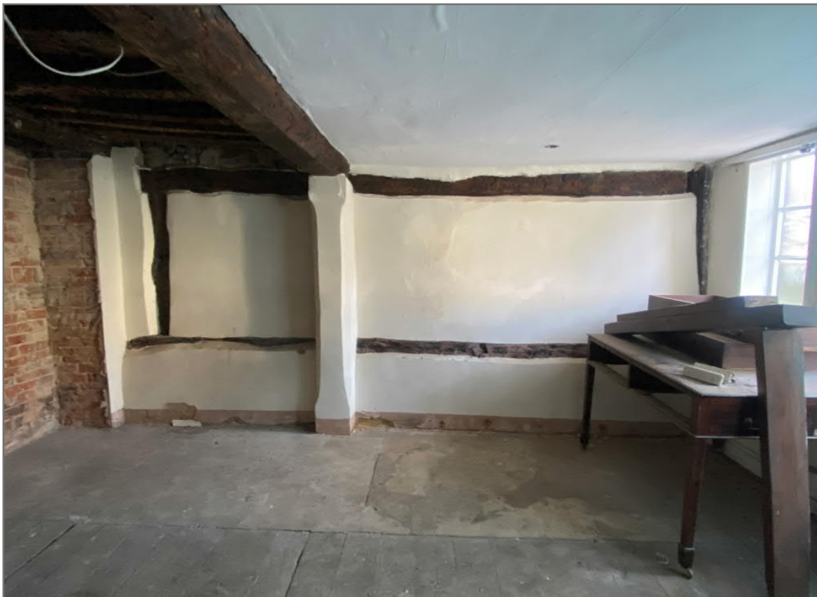
Image 18: View of ground floor room, facing south
