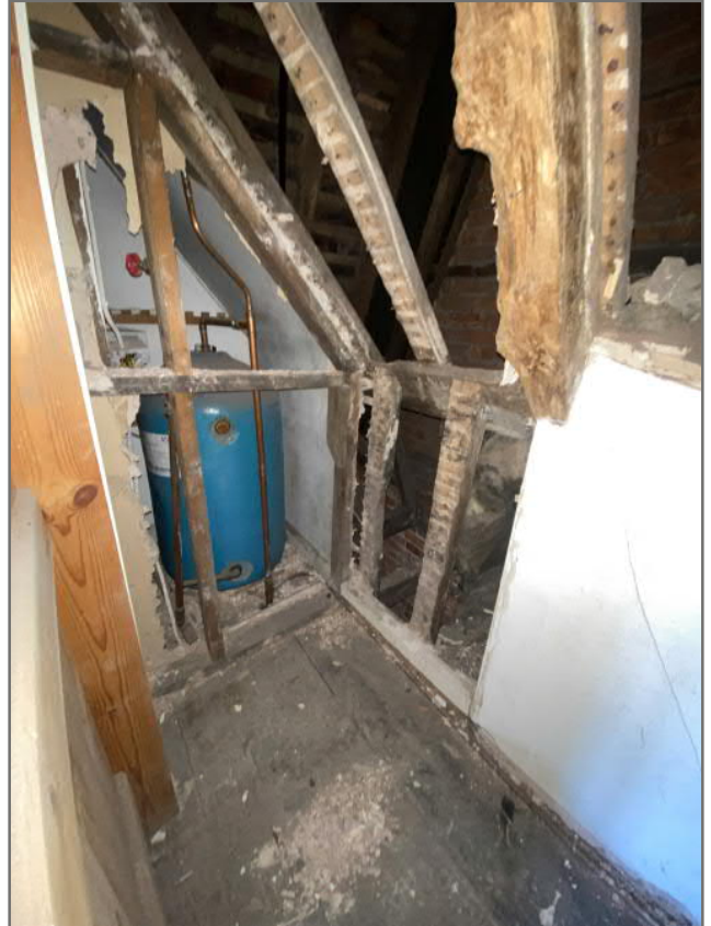
Image 42: Modern internal plasterboard fitting out of southern side of roof - view through to over stairs
