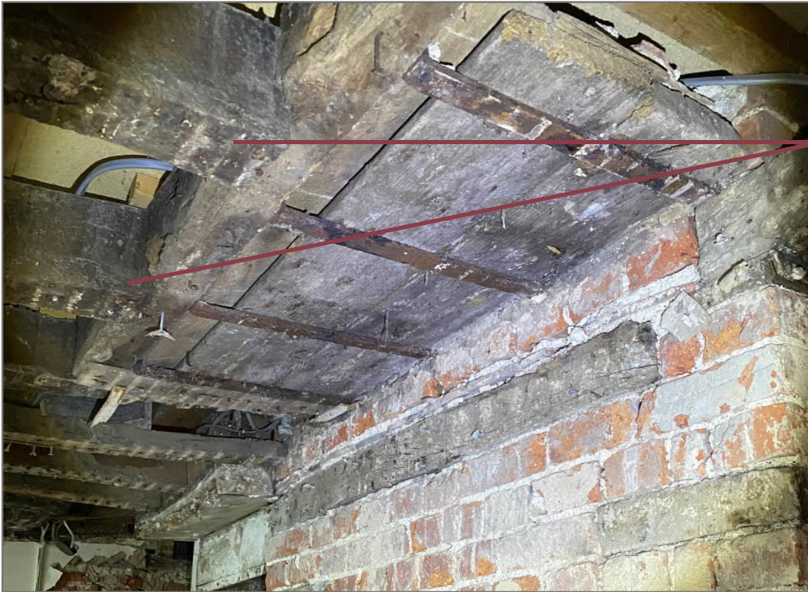
Image 23: View of underside of First Floor hearth
