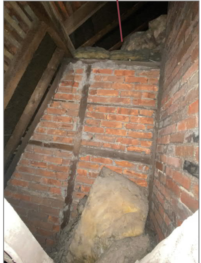
Image 37: View into attic space of east elevation - partywall with No.41
