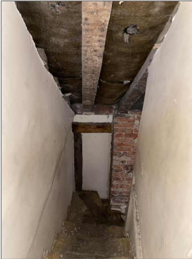
Image 36: View towards east elevation from attic floor
