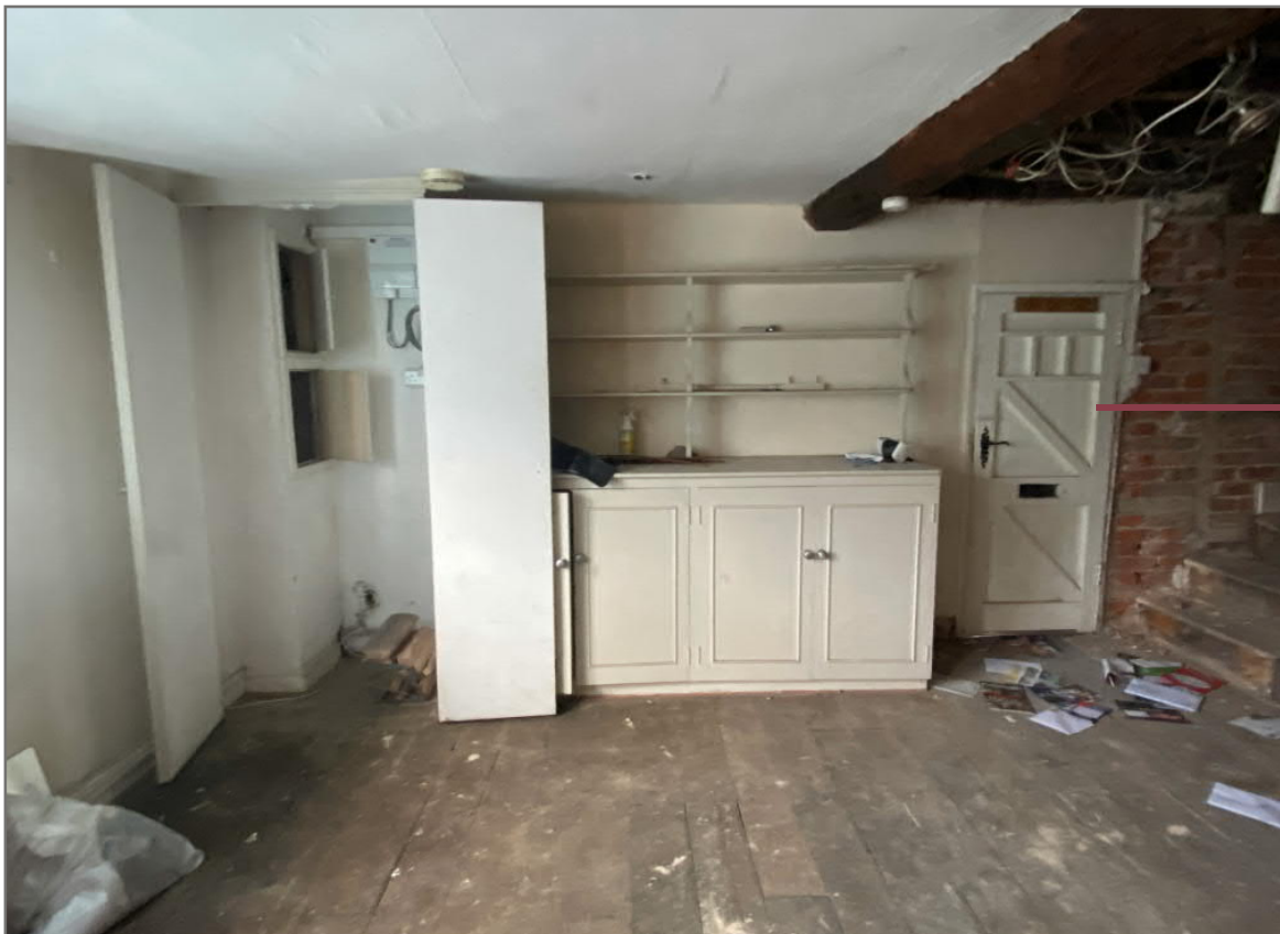
Image 20: View of ground floor room, facing north
