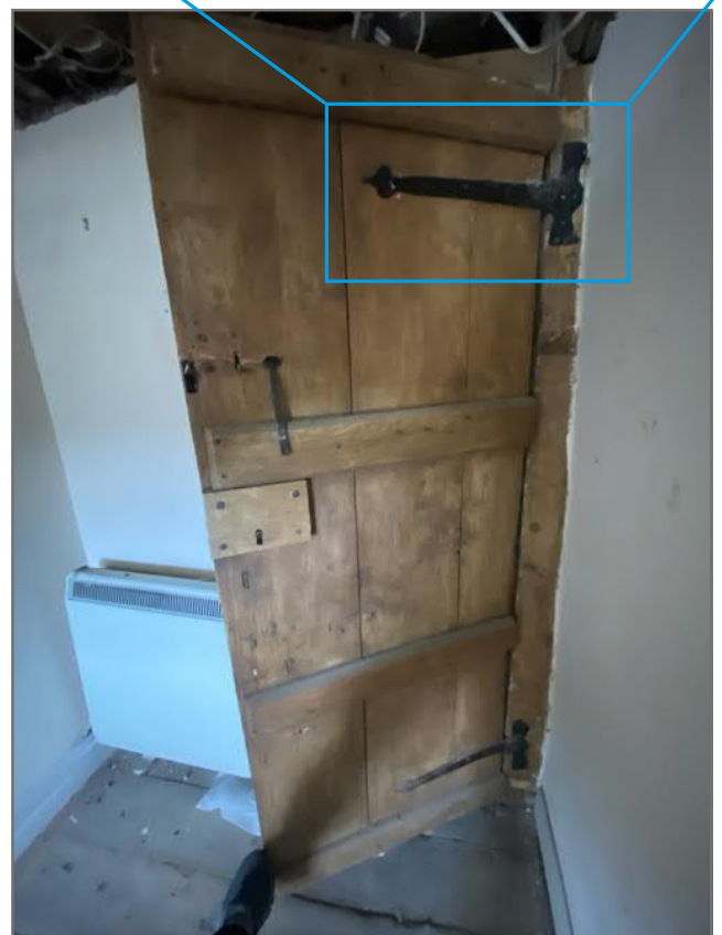
Image 35: Plank and batten door with planks of irregular widths at First Floor - common prior to C19
