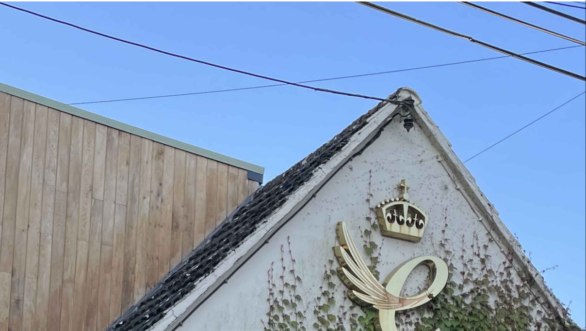
Reference Photo of Existing
