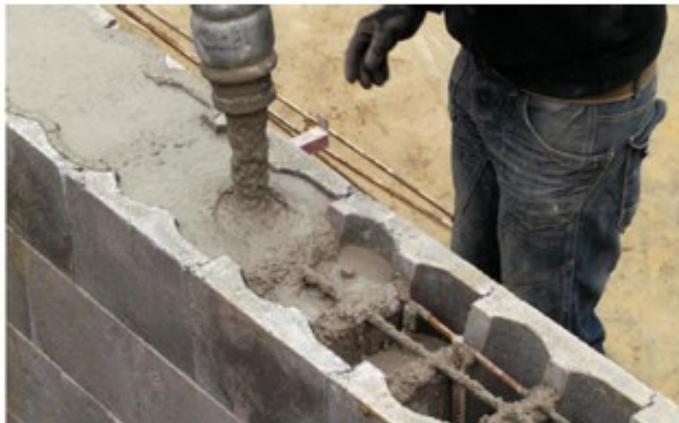
Stepoc hollow block wall with concrete being pumped into pockets
