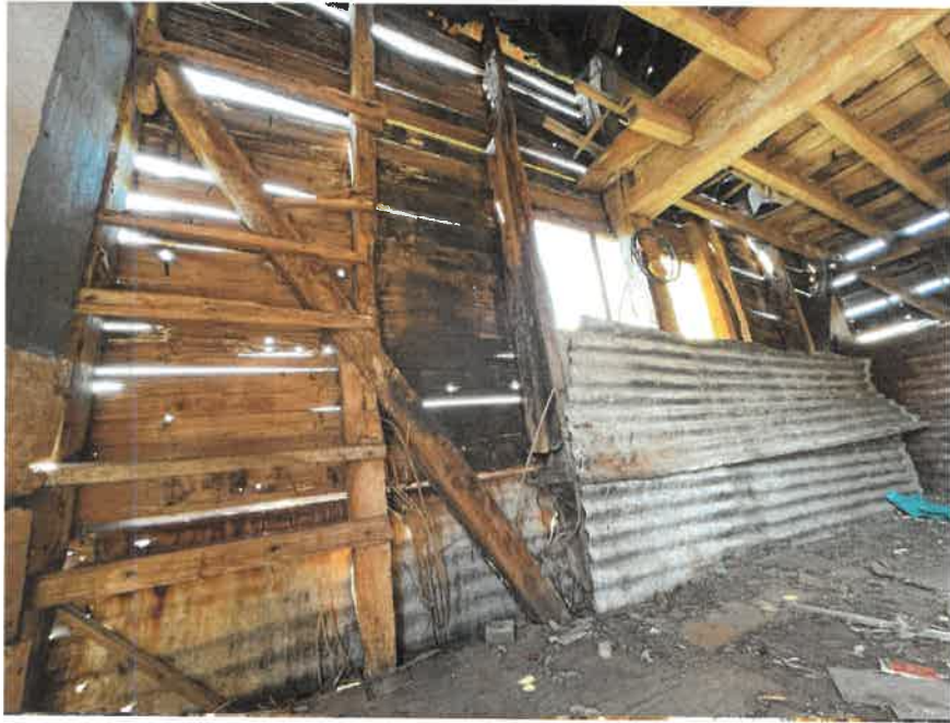
Internal South Wall
