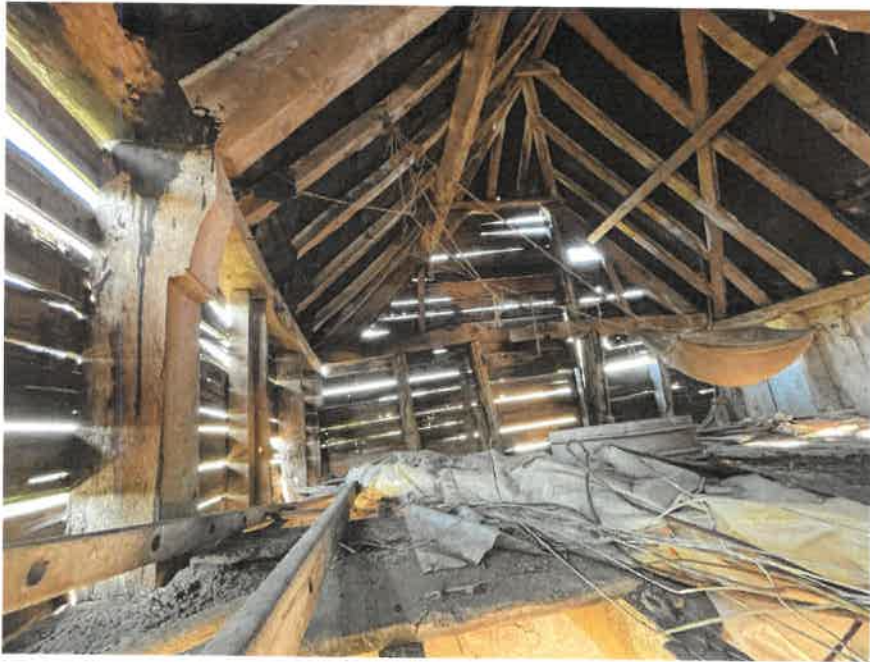
Internal West Gable
