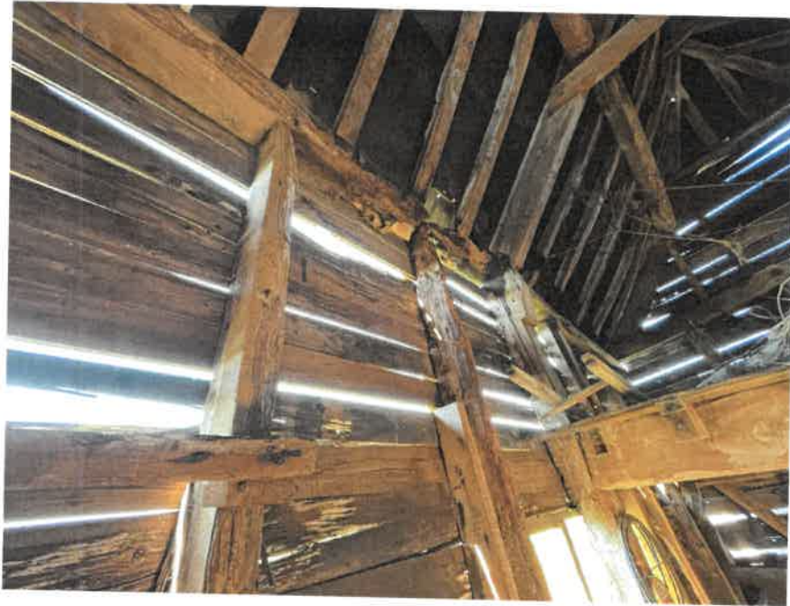
Internal South West
