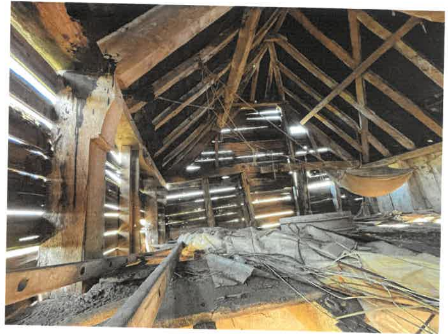
Internal South West
