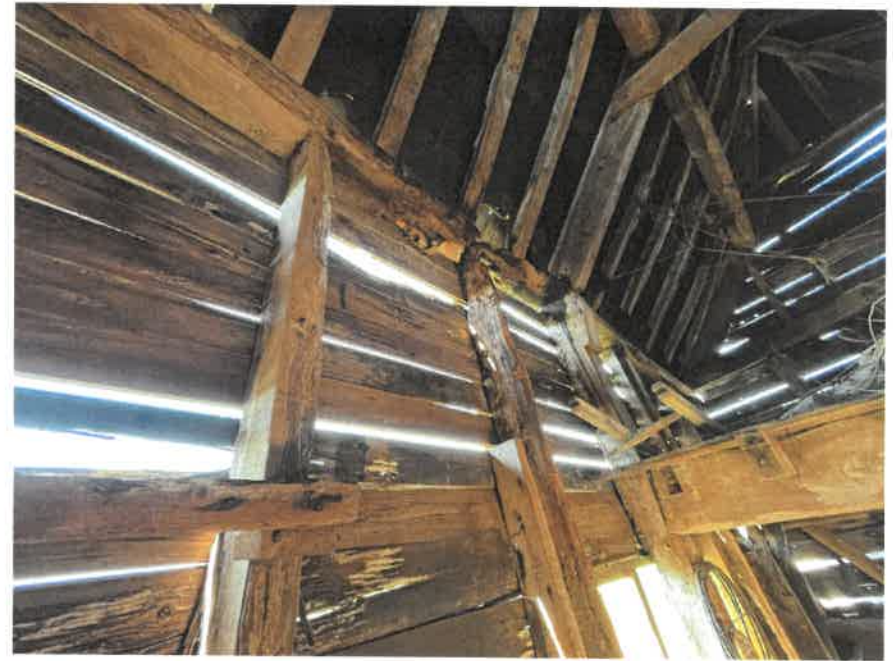
Internal South Wall
