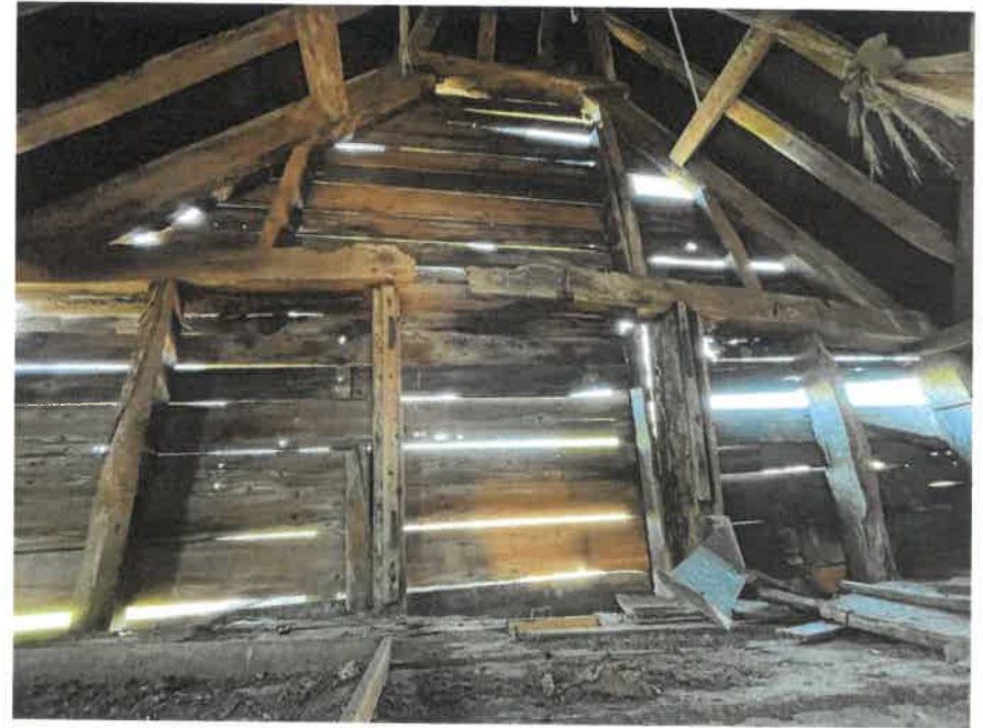
Internal West Gable
