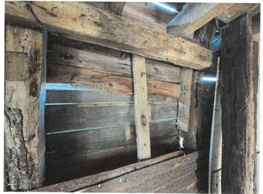
Internal Ground Floor North West
