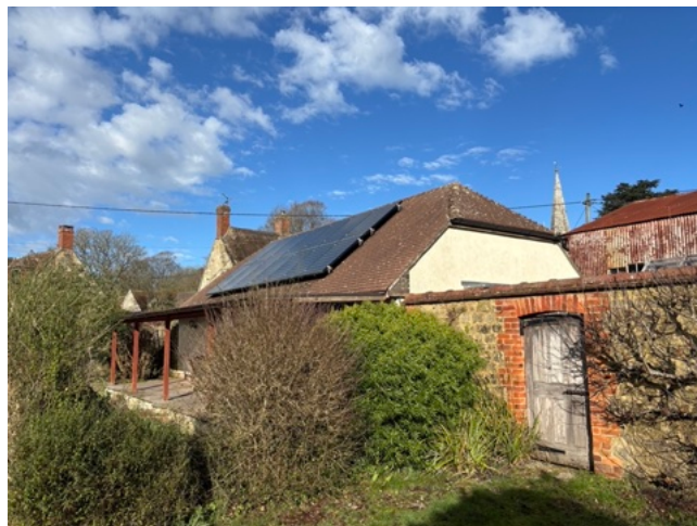
Image 2: Southern corner of the building
