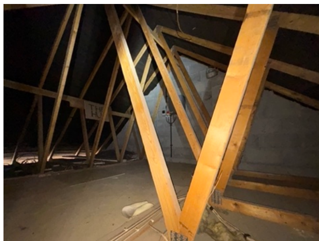
Image 4: Interior of the loftvoid in the Southeastern
