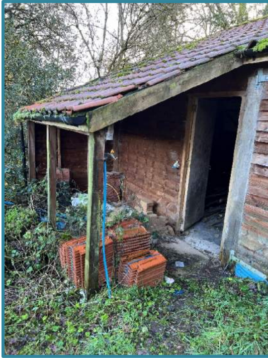
Figure 5 – Lean To Structure
