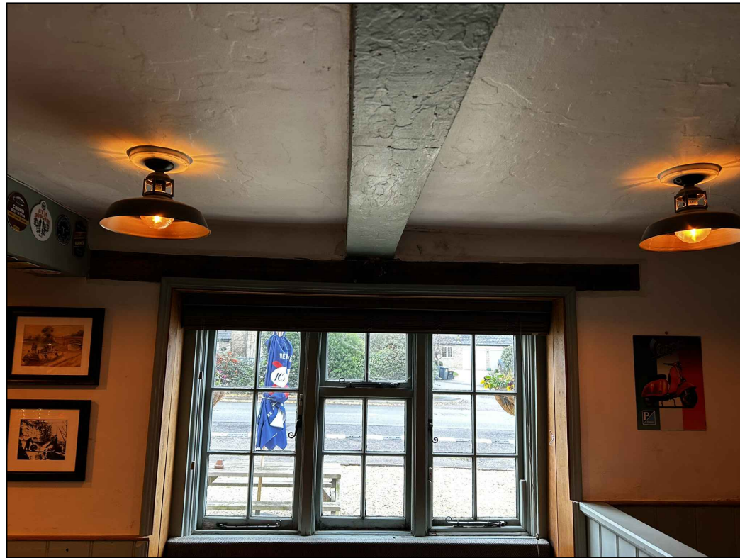
INTERNAL VIEW OF BEAM PRIOR TO INVESTIGATION AND TEMPORARY WORKS
