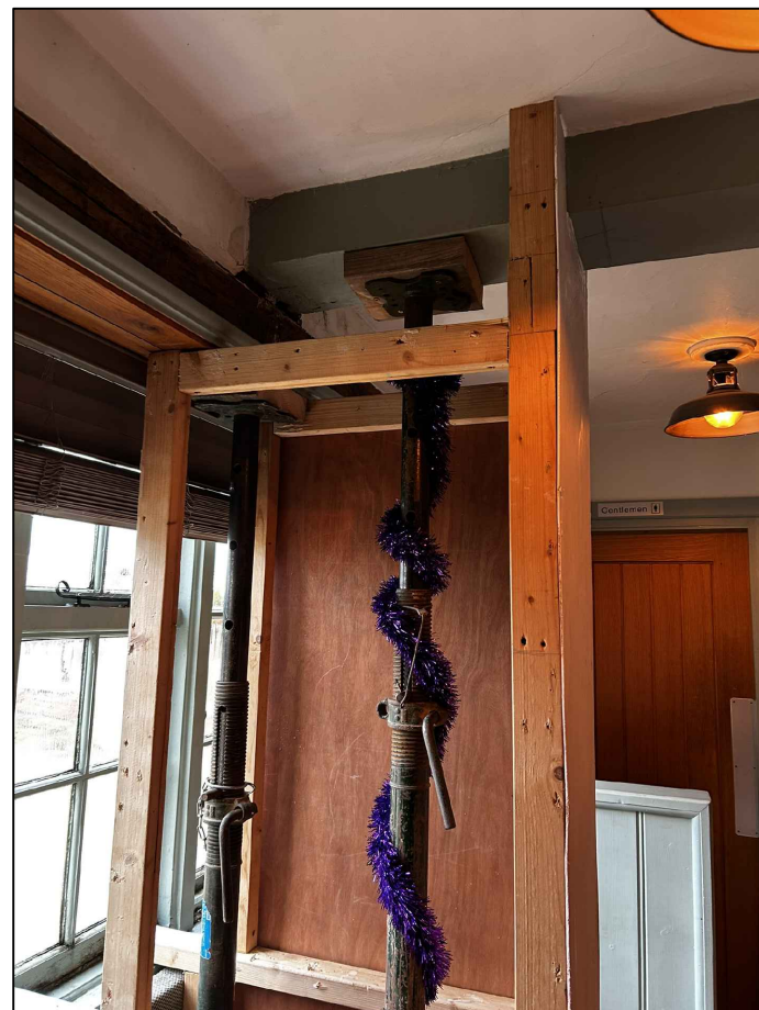
TEMPORARY WORKS INSTALLED
