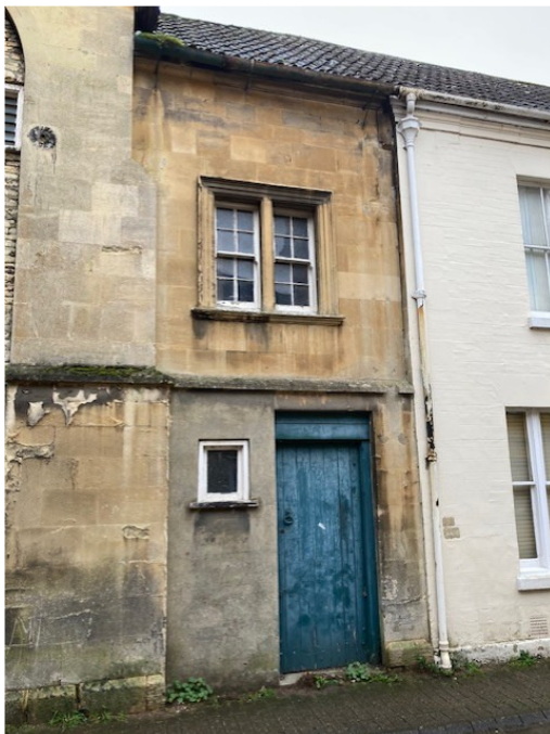
Patford Street elevation lower 2-storey range to the right-hand side built in ashlar limestone
