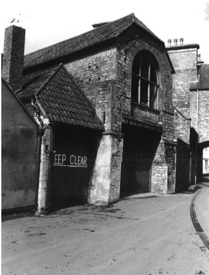
Figure 4 - Photograph taken of the courtyard elevation c1986 (Historic Englands Listing description)
