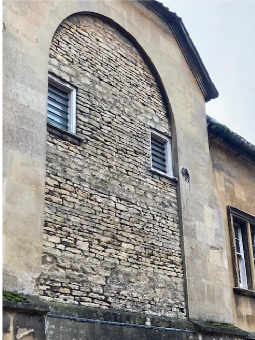
Patford Street Elevation ashlar full height round-headed archway with rubble between
