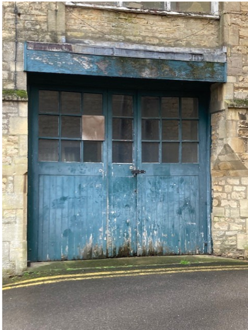
Large doors to the courtyard elevation
