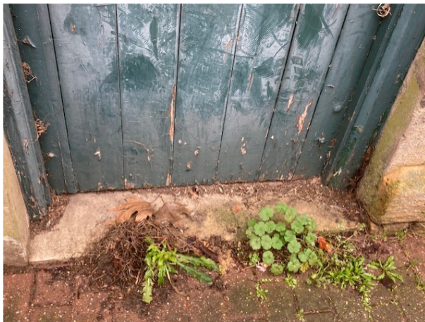
Single pedestrian door on Patford Street
