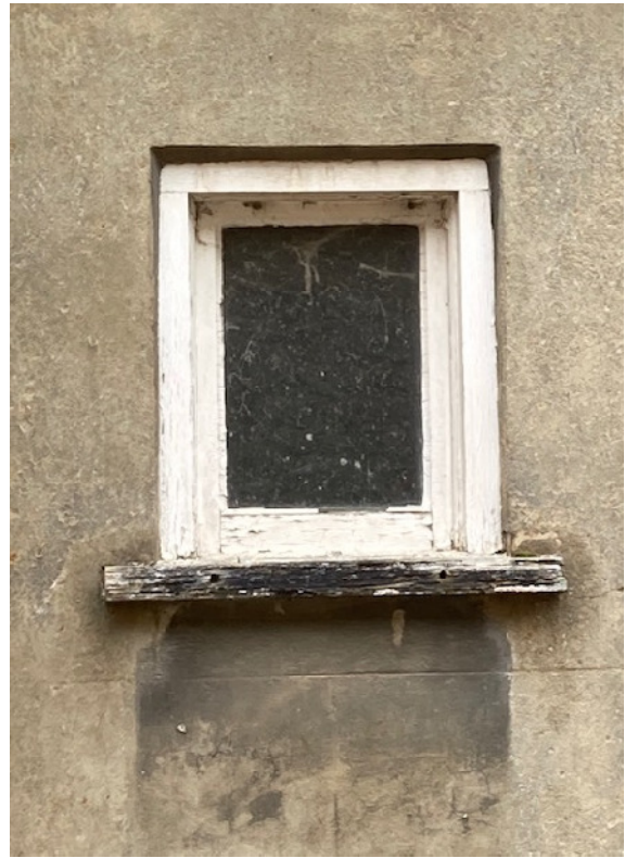
Small window on Patford Street elevation
