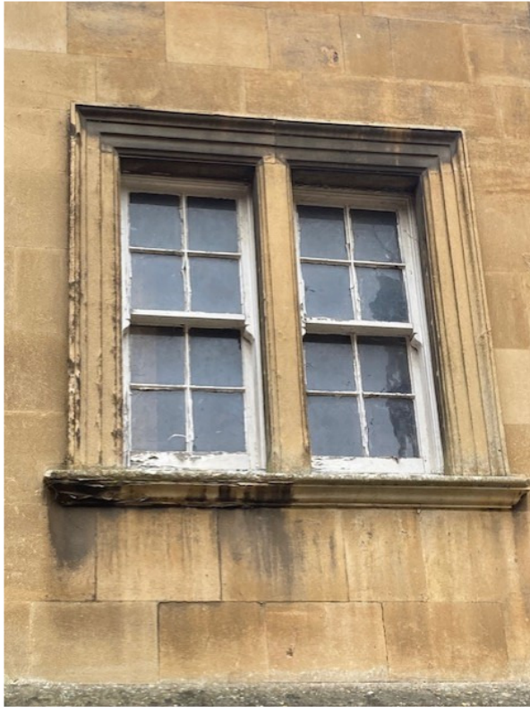
Window facing onto Patford Street
