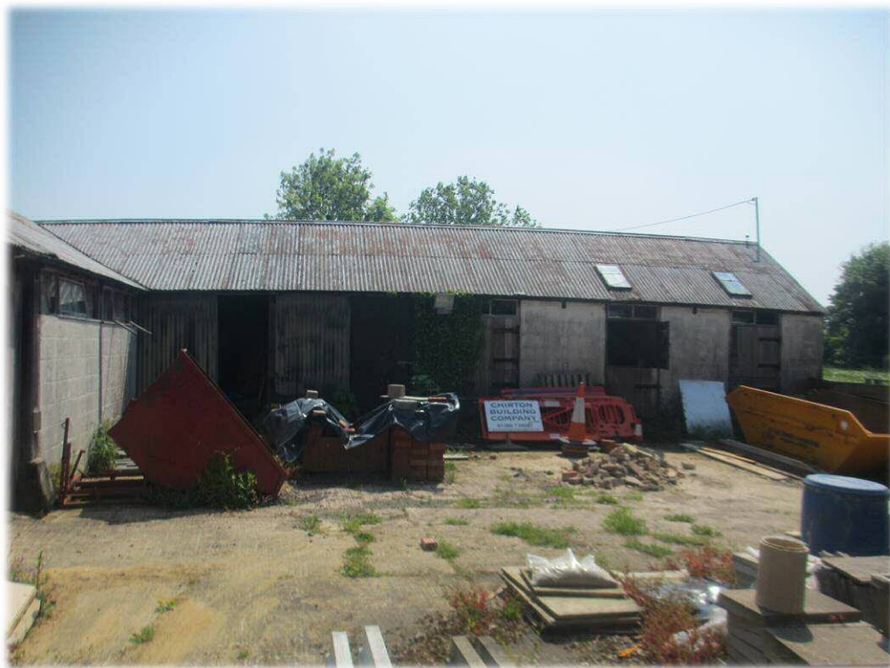
Building 1b exterior
