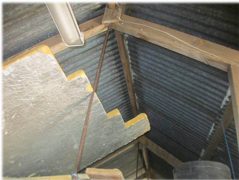
Building 1b roof structure
