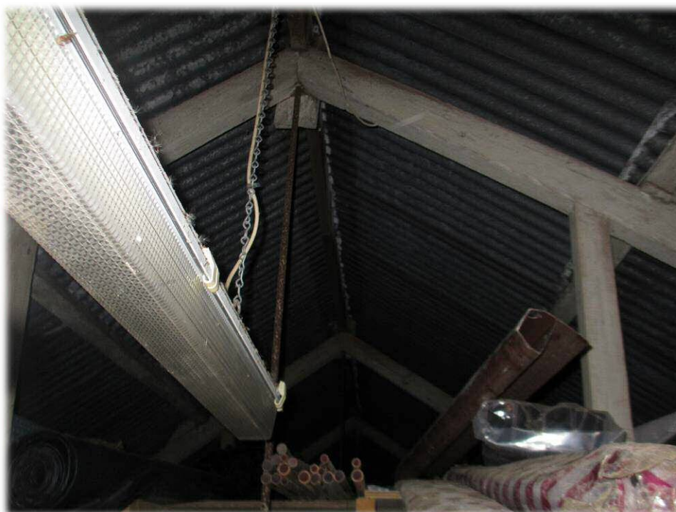
Building 1a roof structure
