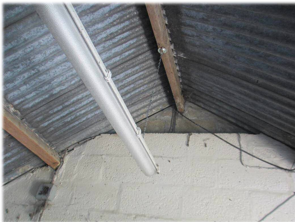
Building 1b southern gable end blockwork wall
