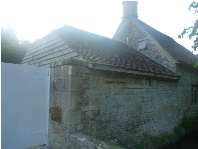
Fig 3: Garage at Fitz House, showing stone blockwork, timber cladding and clay roof tiles.
