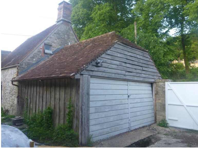
Fig 2: Garage at Fitz House, showing timber cladding and clay roof tiles.
