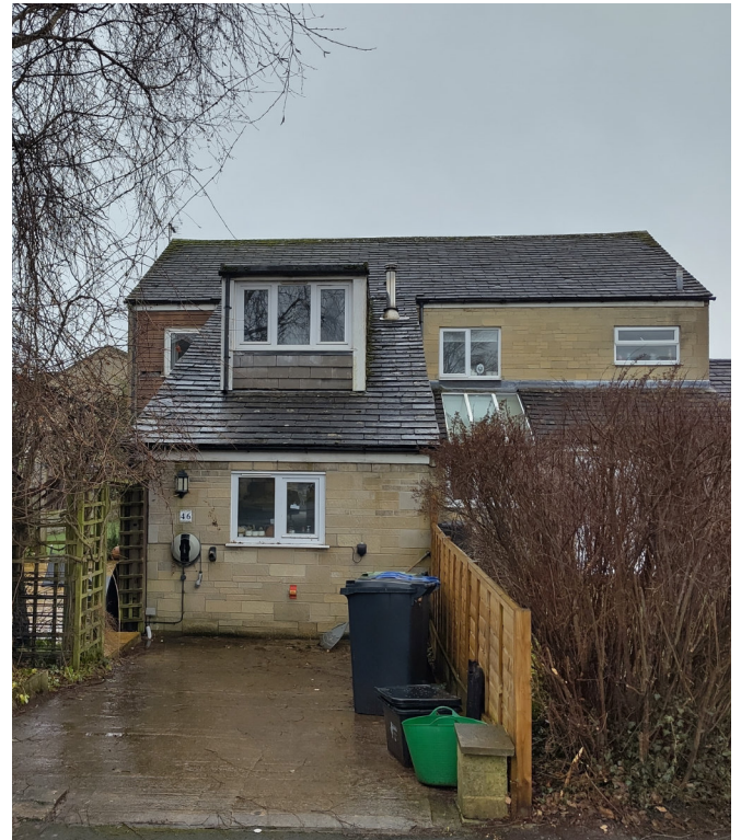
View of the front (street) elevation
