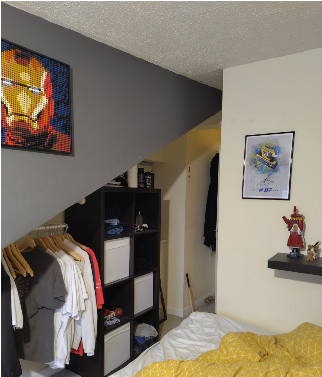
The low areas under the roof have limited usable space
