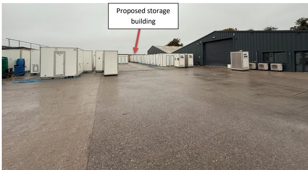
Figure 3 - Current photograph of the existing site showing position of proposed building
