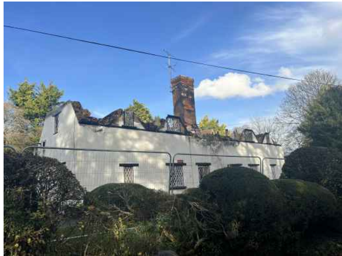
Front (south) view
