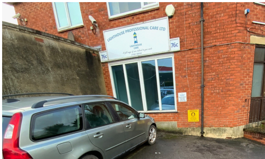
Figure 2 South-East Window to be replaced
