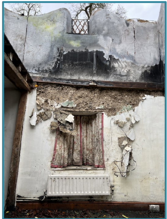
Figure 11 – Window Head South Elevation (West End)
