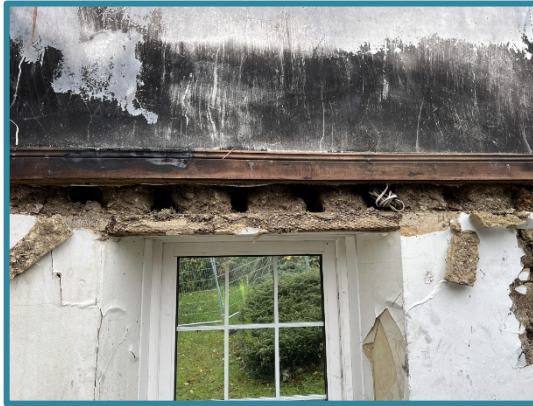
Figure 12 – Post Holes in Cob
