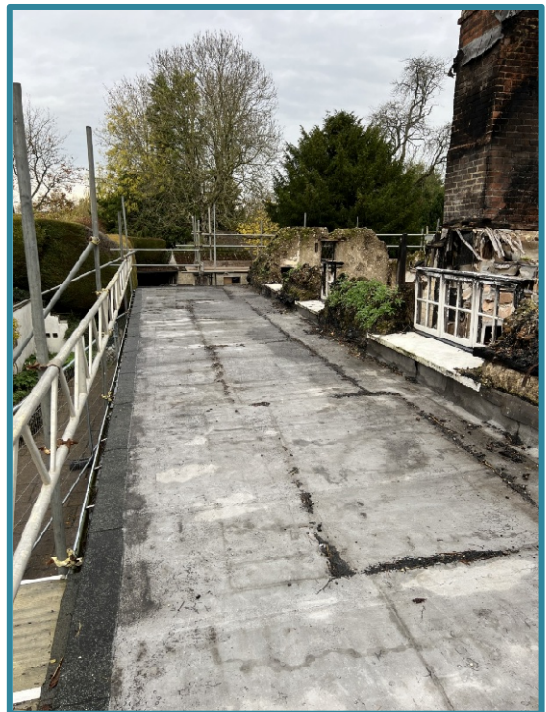
Figure 15 – North Appendage Roof
