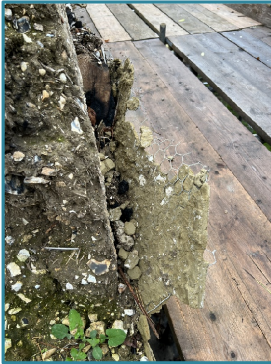
Figure 6 – Reinforced Cement Render
