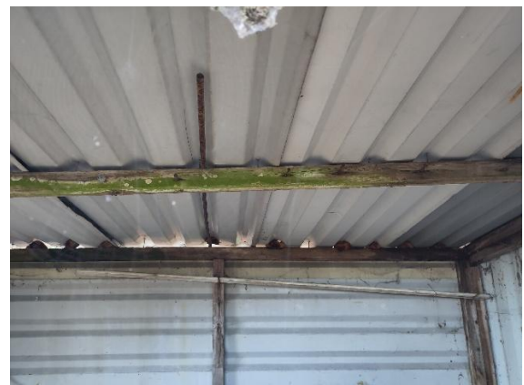
Figure 12: Internal of building B1
