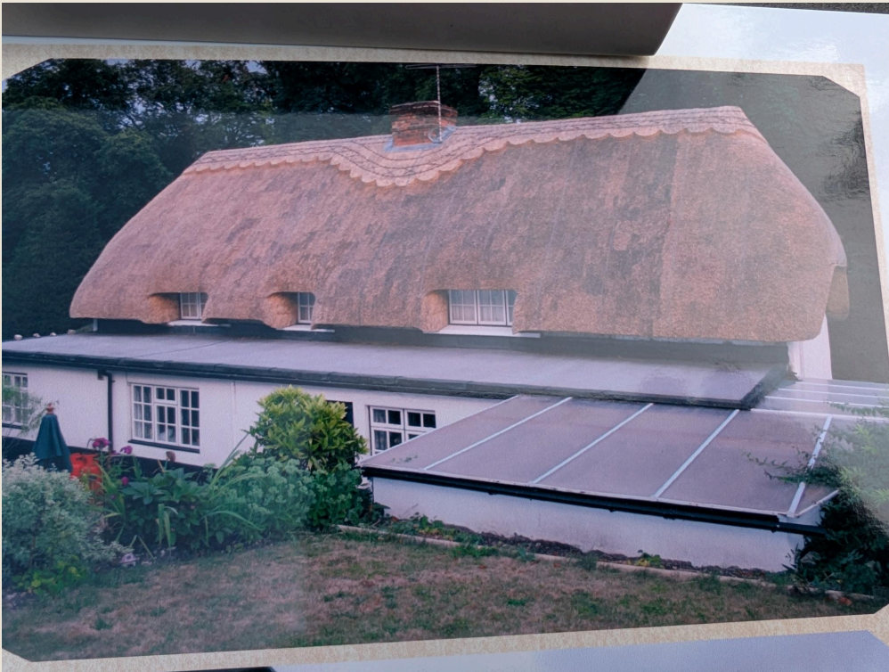
Figure 6 – Rear view of Hackthorne Cottage facing South, pre-fire
