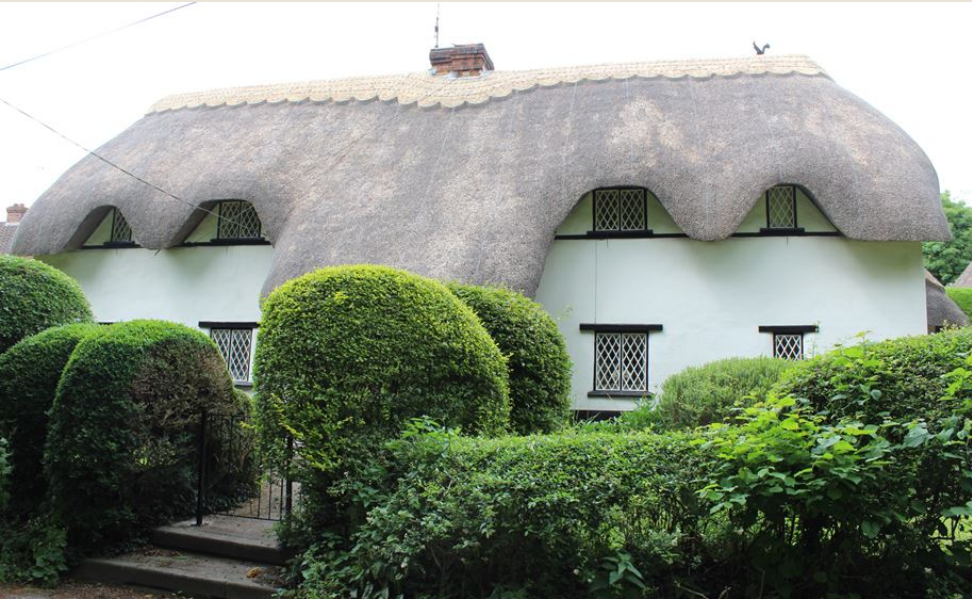
Figure 3 – Hackthorne cottage front elevation, facing North, pre fire
