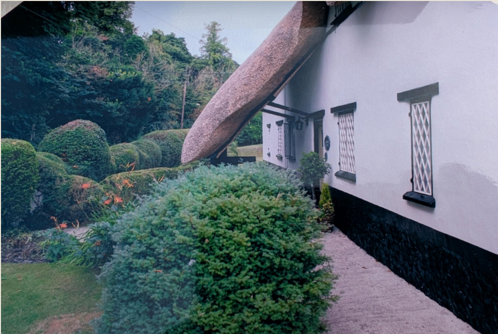
Figure 5– Thatch overhang covering well and front entrance, to be restored
