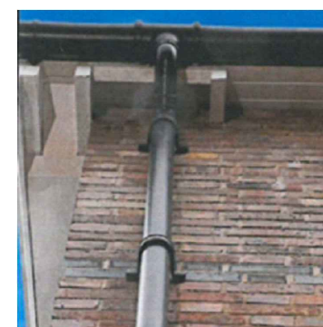
PROPOSED RAINWATER GOODS, FASCIA AND SOFFIT BOARDS
