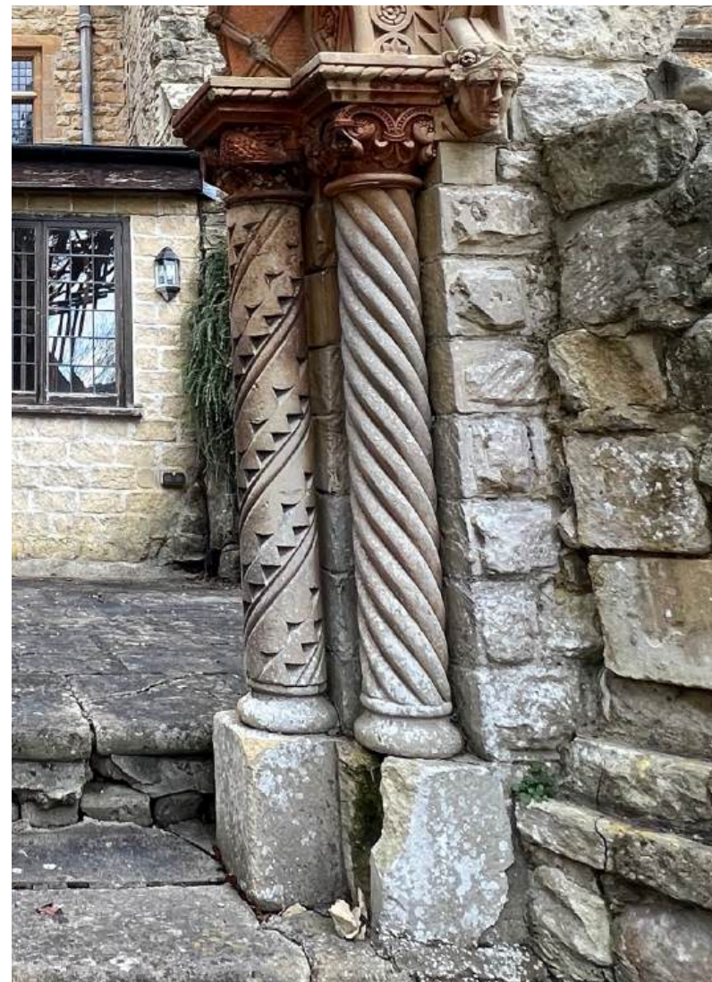
Figure 5 Southern jamb, west side.
