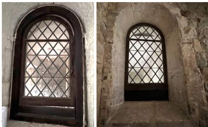
Figure 72 Sub ante room, interior & (former) exterior of window in north wall.
