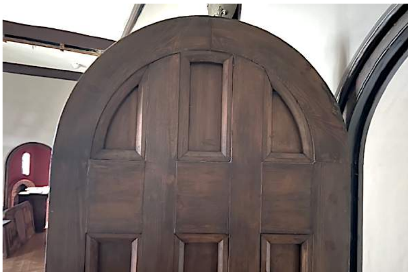
Figure IO9 Door between Dining Room & back stair.
