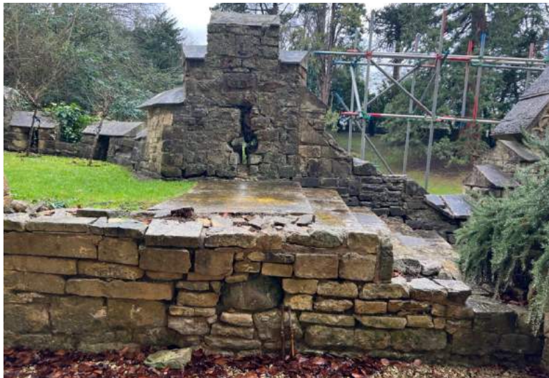
Figure 82 View from east; the tunnel runs directly beneath the paved stone landing, with light visible through the masonry in the foreground.
