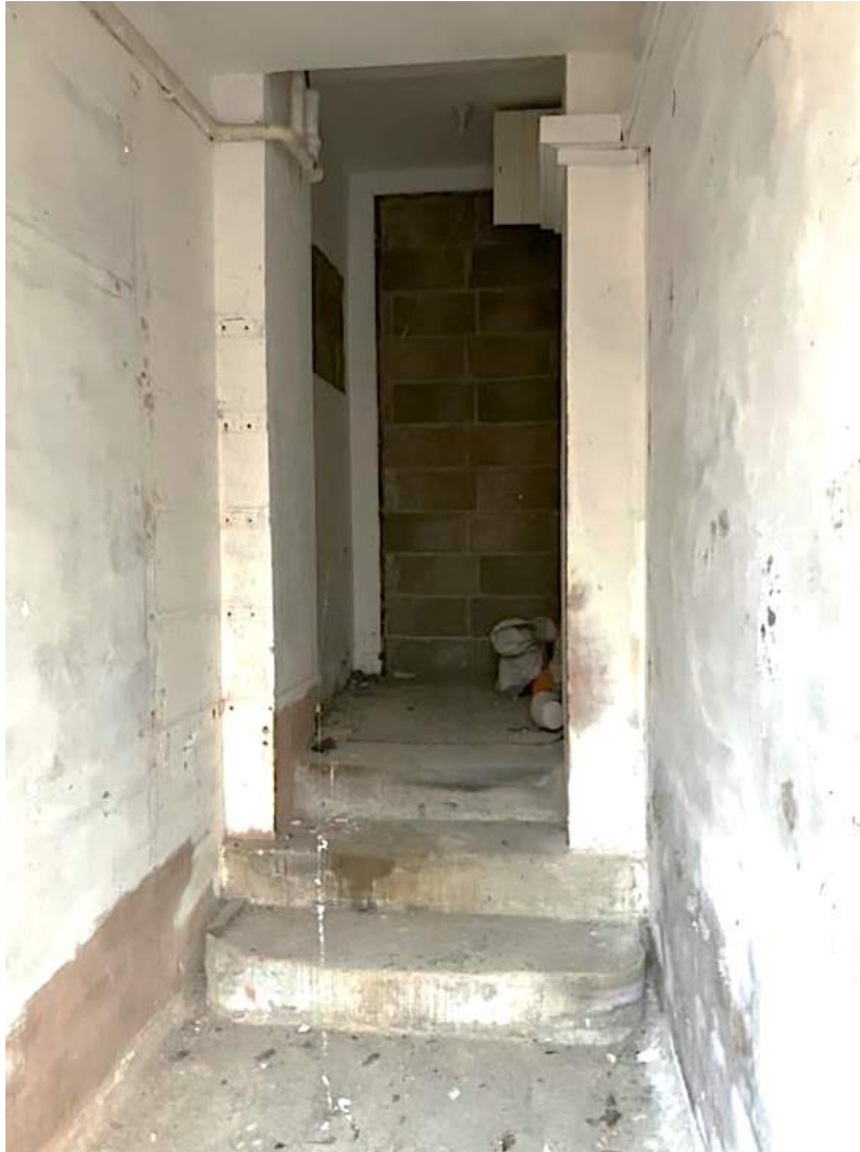
Figure 92 Former northern service entrance.
