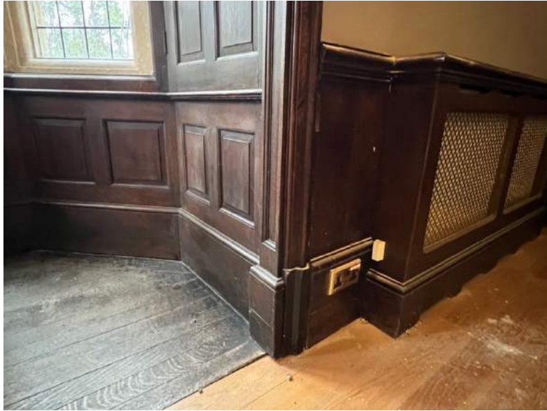
Figure 104 Dining Room bay, detail of linings.
