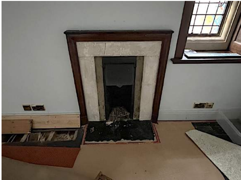
Figure 175 Bedroom (above Gallery), fireplace.
