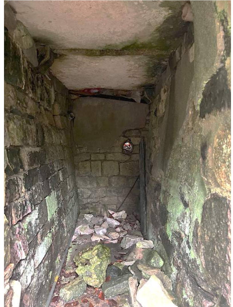
Figure 83 View into tunnel, the underside of paving stones form the ceiling, & light visible through the blocking.
