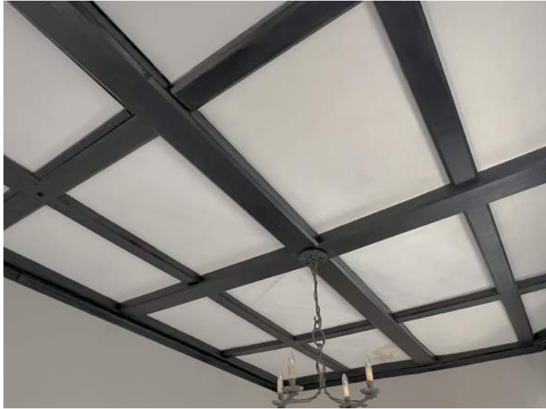
Figure 188 Bed Room over Drawing Room, ceiling.
