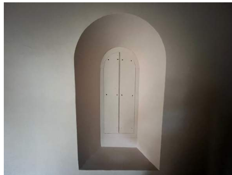
Figure 170 Former window in the east wall of the Boudoir .
