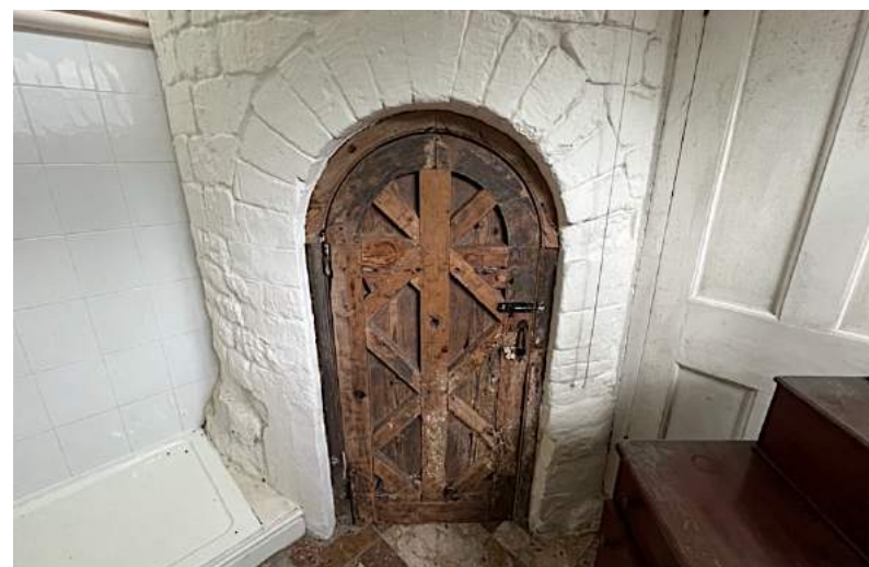
Figure 155 Door at the foot of the turret stair.
