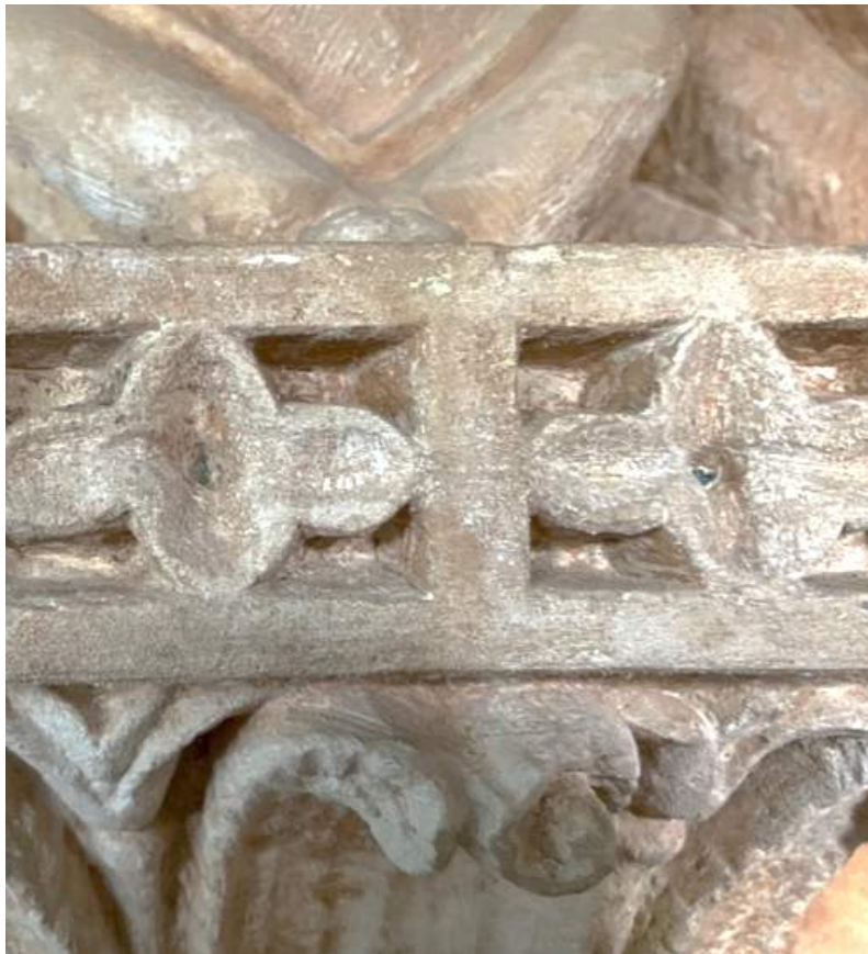
Figure 132 Detail of the abacus of the eastern jamb of the arch.
