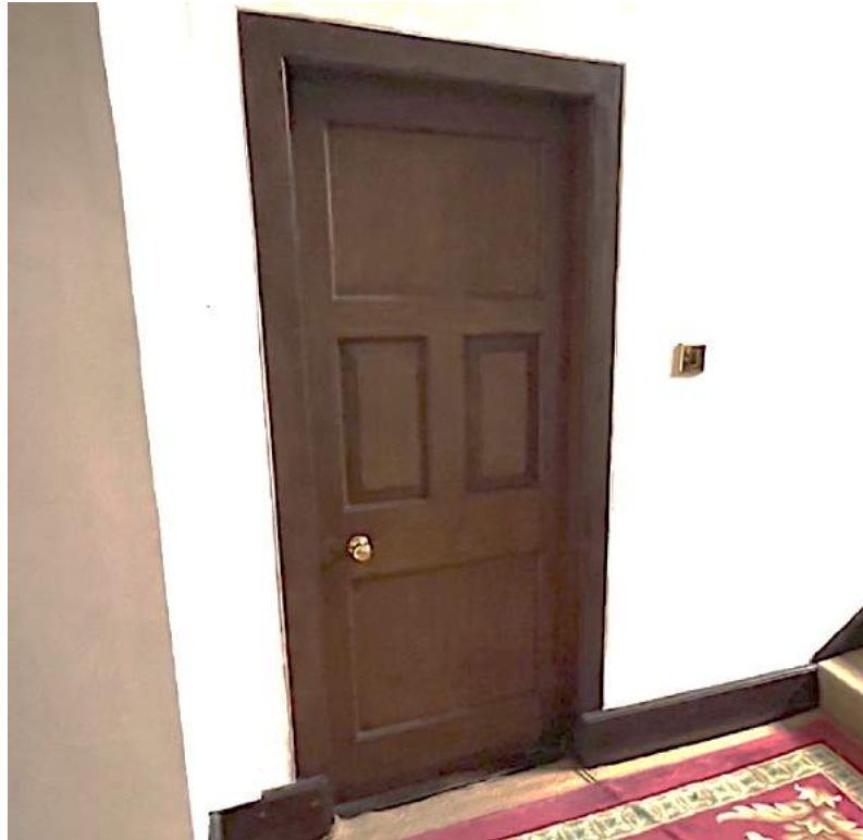
Figure 151 Rich-phase door & architrave to the Cloak Room .
