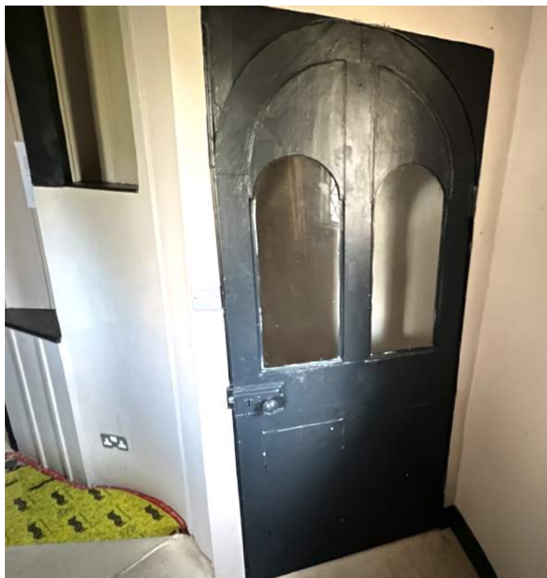
Figure 194 Door to stair down to Secret Chamber/Museum Room .
