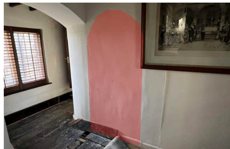
Figure 179 Passage & stair, opening to Rich-phase extension (left) & blocked door to Bedroom (above Gallery) to right.
