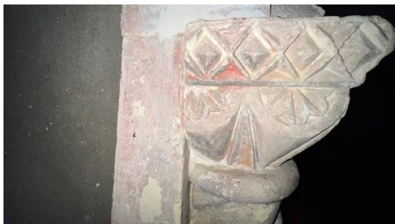
Figure 114 Detail of right-hand colonette showing evidence of polychromatic decoration.
