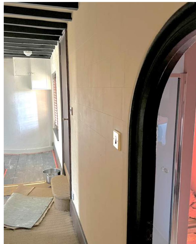
Figure 197 Corridor & partition to west of Front Bed Room.
