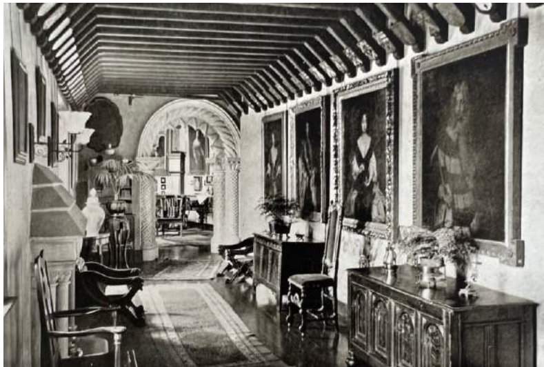
Figure 128 Gallery facing north, 1914 sales particulars (Historic England Archive, SC01216).
