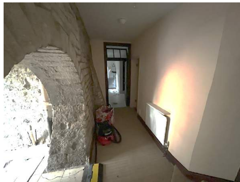
Figure 89 Corridor, facing north.
