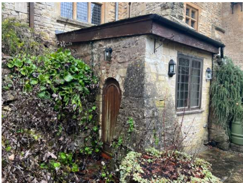
Figure 84 Northern store, from the north-west.
