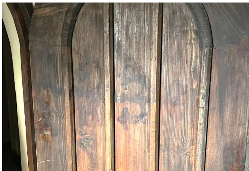
Figure 73 Sub ante room, detail of door in north wall (outside face), showing scars from now-removed decorative ironwork.
