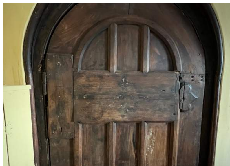
Figure 126 Detail of door from gallery to turret stair.
