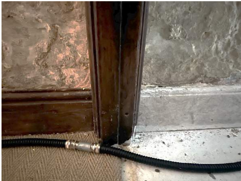
Figure 90 Corridor, details of skirtings to either side of modern dividing wall: modern skirting to south/left; historic (Rich phase) skirting to north/right.
