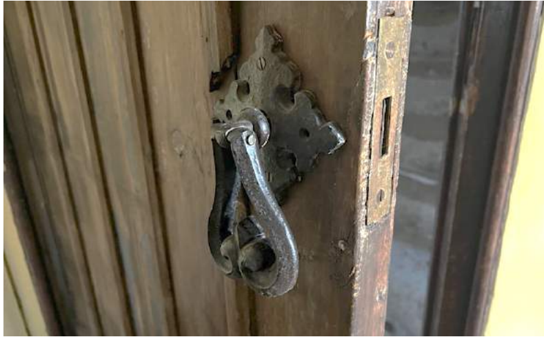
Figure 127 Detail of handle on door to turret stair.
