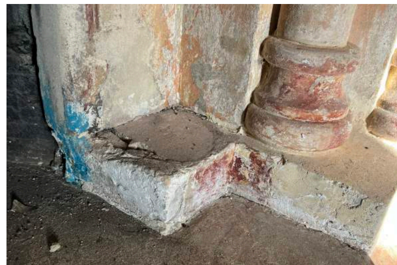
Figure 184 Detail of fireplace; base of right jamb.
