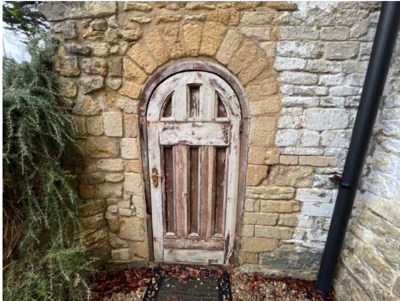
Figure 86 Northern store, south door.
