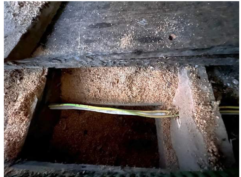
Figure 172 Boudoir floor construction, showing thick layer of sawdust pugging on pugging boards between the joists.
