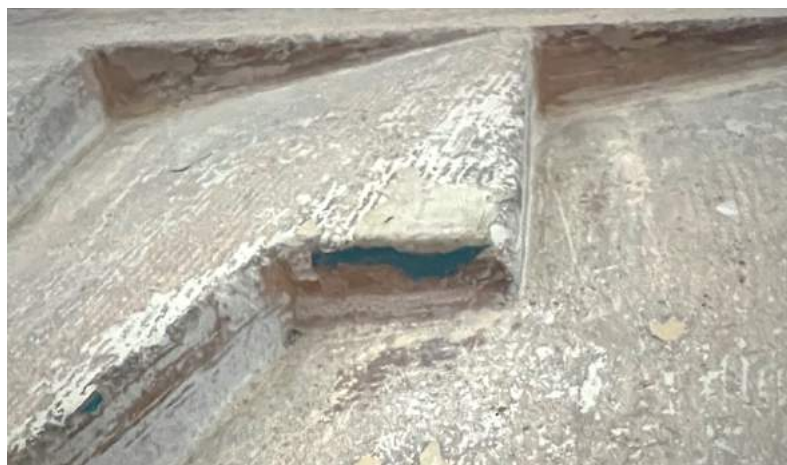
Figure 125 Fragment of blue paint surviving on Gallery fireplace.
