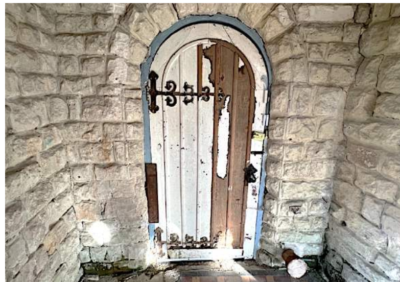
Figure 149 Fernery, door at southern end (to former Conservatory ).
