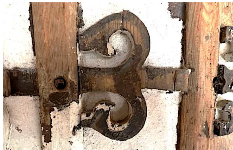
Figure 150 Conservatory door, detail of applied timber strap hinges.
