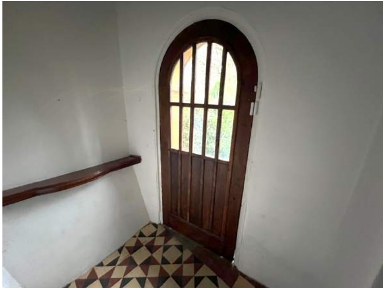
Figure 100 Lobby (garden entrance).
