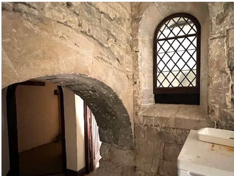
Figure 88 Northern store, entrance from adjacent corridor.
