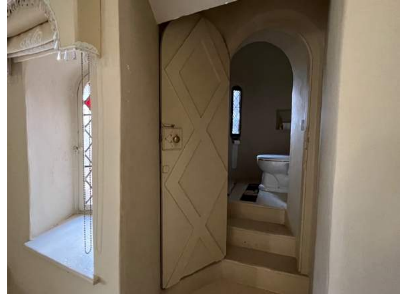
Figure 191 Door to turret closet.
