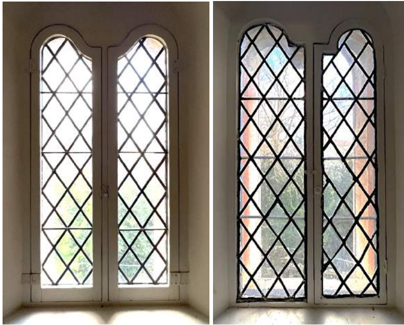
Figure 190 Detail of windows.
