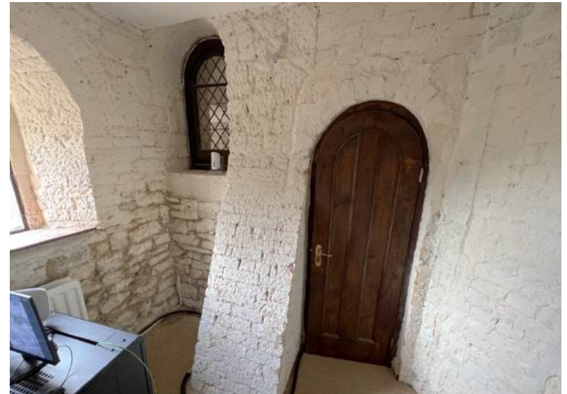
Figure 71 Sub-ante room, north wall.
