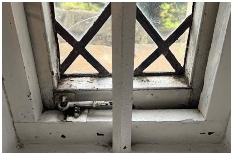
Figure 153 Detail of timber casement.
