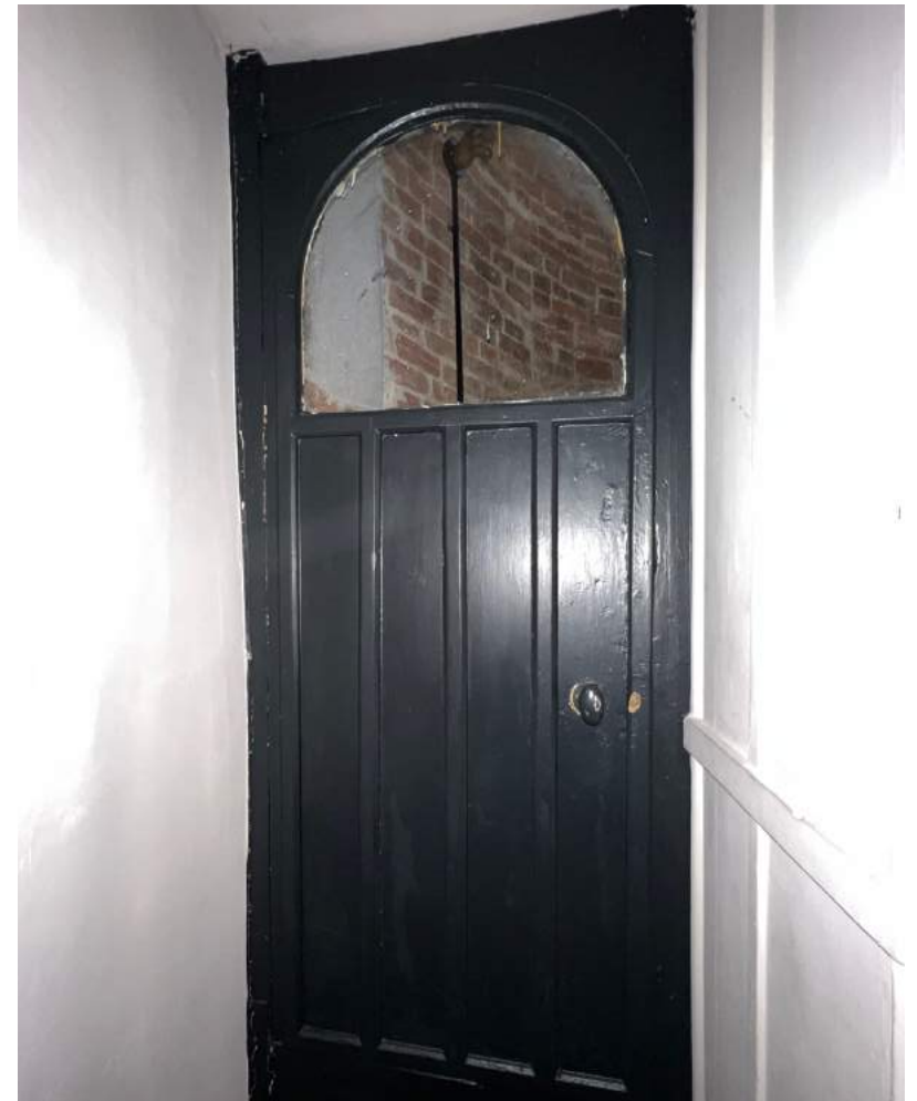
Figure 204 Door to Top Bed Room in Ivy Tower.
