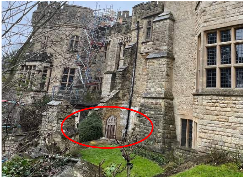
Figure 79 West front, location of lost wall which concealed the now-removed store.
