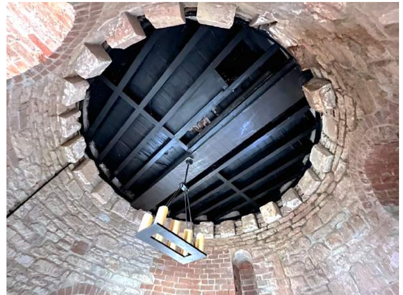
Figure 206 Top Bed Room in Ivy Tower, ceiling.
