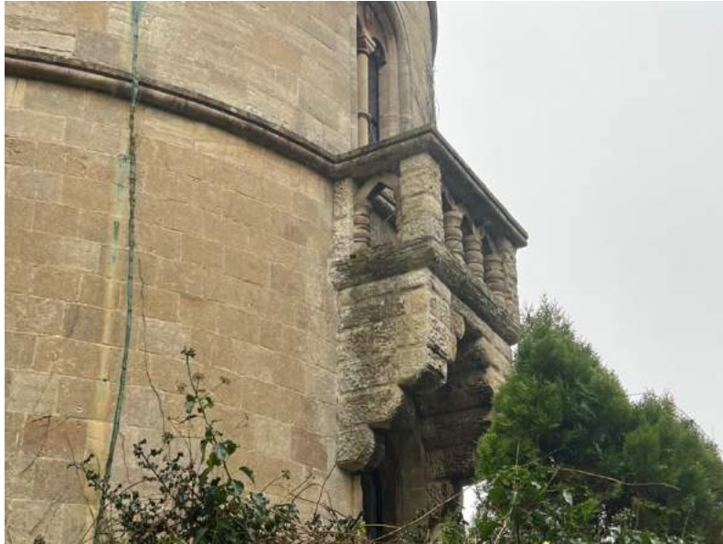
Figure 165 South tower, showing decorative balcony placed in front of pre-existing (albeit enriched) window.
