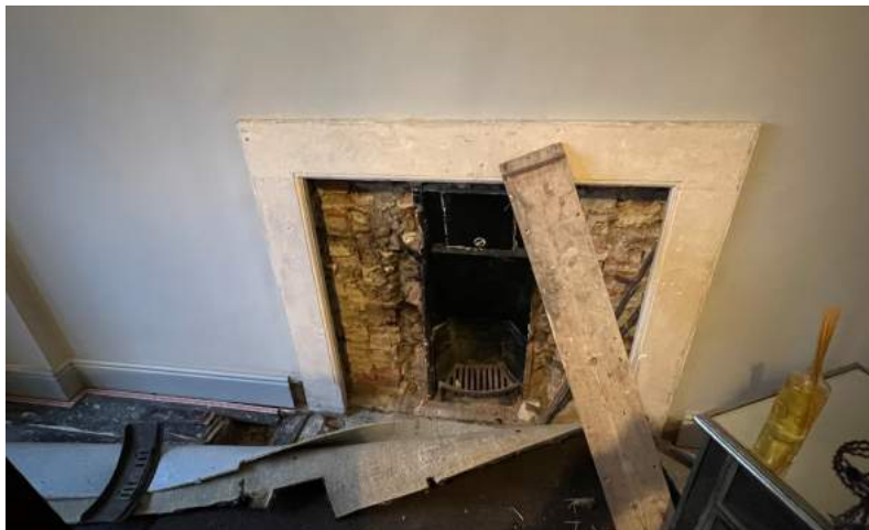
Figure 203 Southern bedroom above Billiard Room, detail of fireplace.
