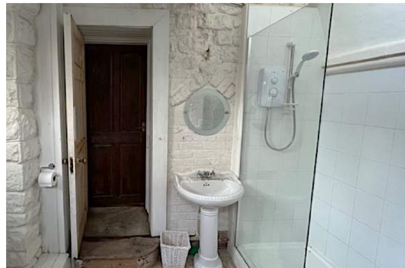
Figure 154 Modern bathroom door, with blocked opening to right.
