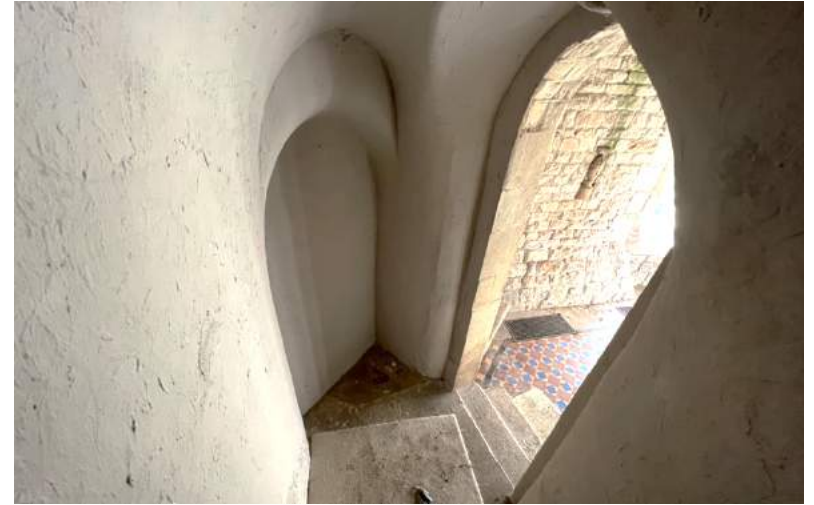
Figure 138 Former door from the Drawing Room to the Ivy Tower & Fernery .
