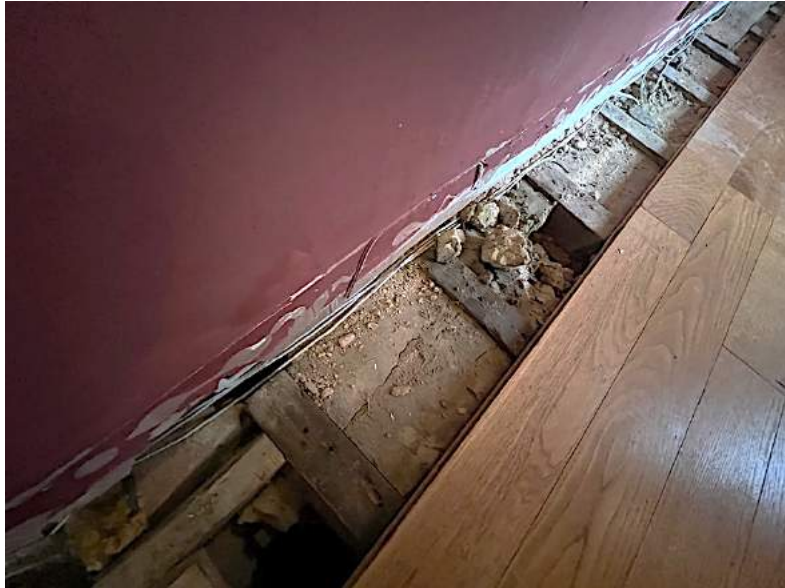
Figure 116 Pugging beneath Ante Room floor.
