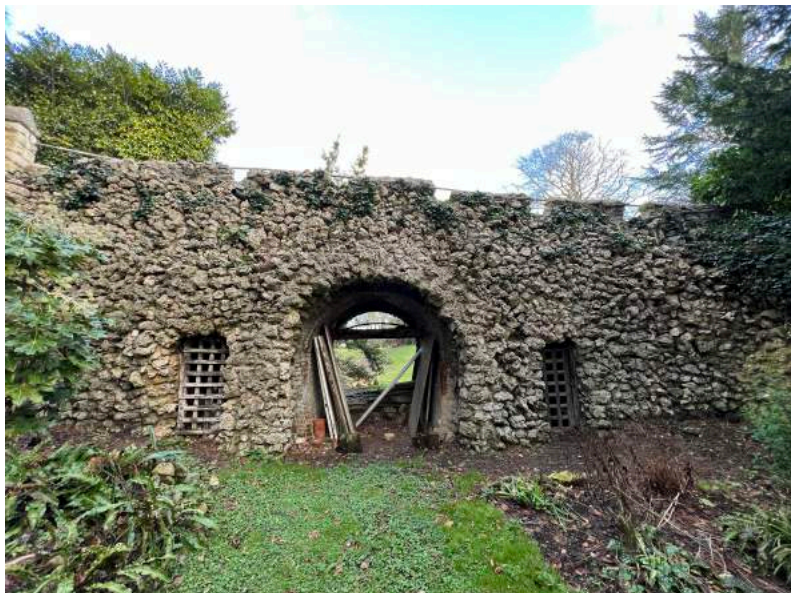
Figure 213 Bridge, south-west elevation.
