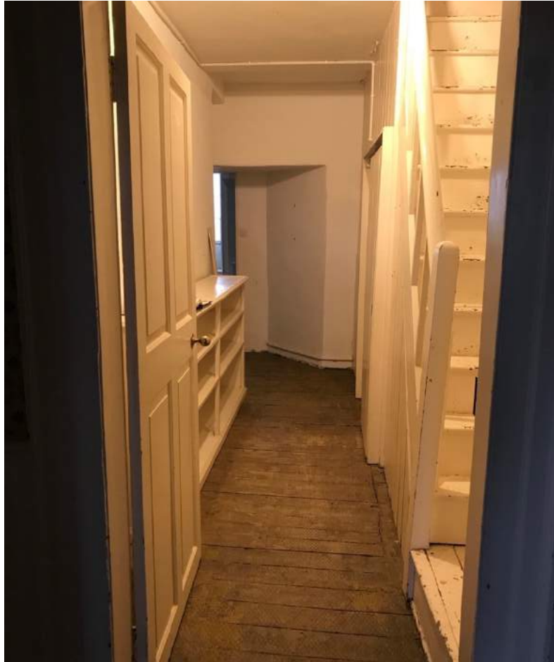
Figure 26O Simple 19 th -century roof access stair from the second floor of an early-18 th century country house in Shropshire.
