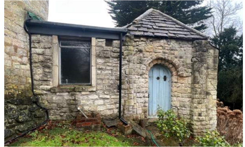
Figure 254 Window to room behind Fernery .
