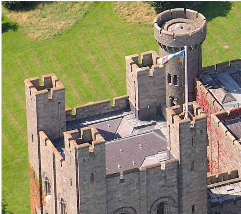
Figure 269 Penrhyn Castle, Bangor, Thomas Hopper, 1822-37; roof of keep showing door from turret & walkway behind the parapet.
