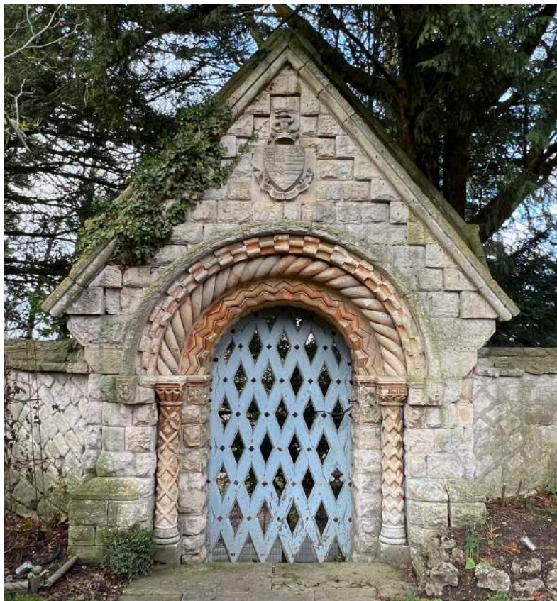
Figure 226 Northern gate, inside face.
