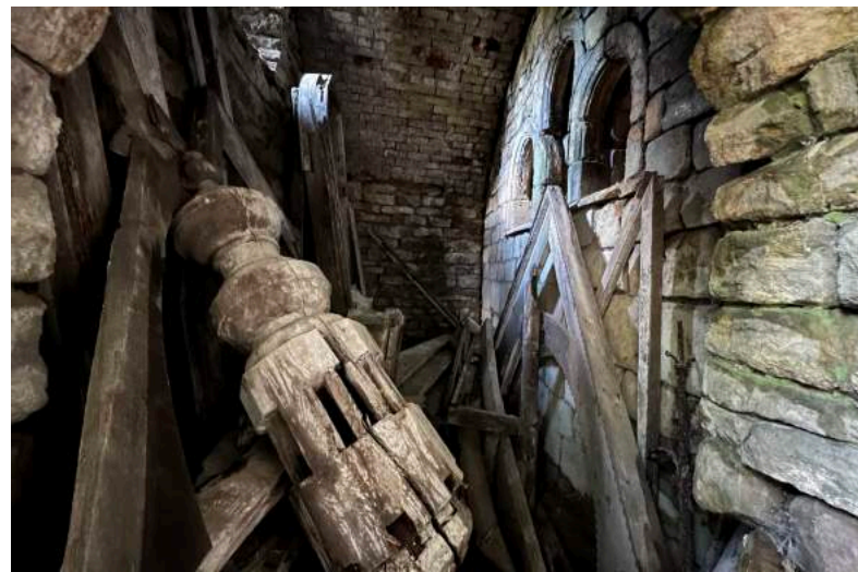
Figure 214 Bridge, original north-east elevation, from within later addition (showing stored structure from the former Conservatory ).
