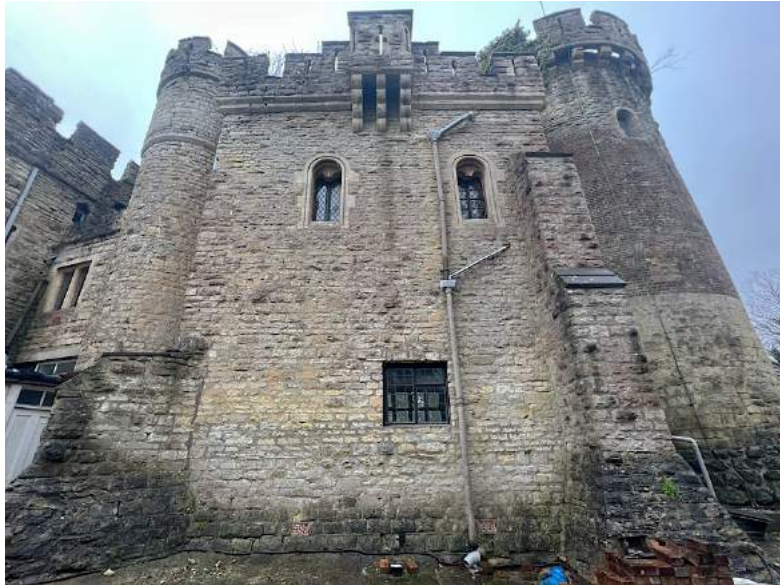
Figure 247 East elevation, showing modern window to rear of Drawing Room .
