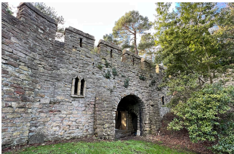
Figure 216 Bridge, current north-east elevation.
