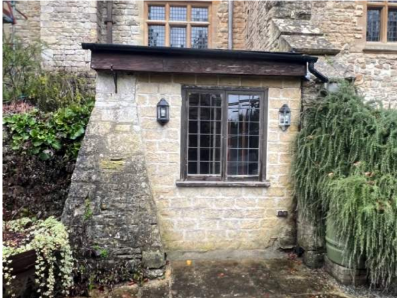
Figure 249 Northern store/boot room, west front.
