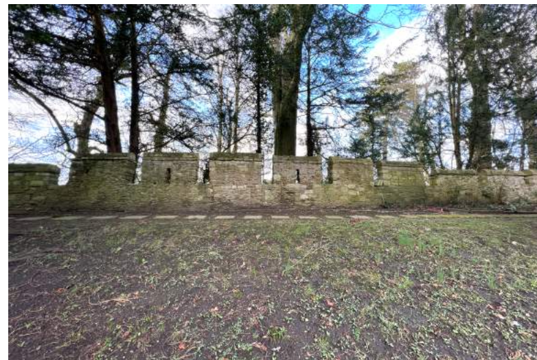
Figure 229 Six taller merlons, with two arrow loops.
