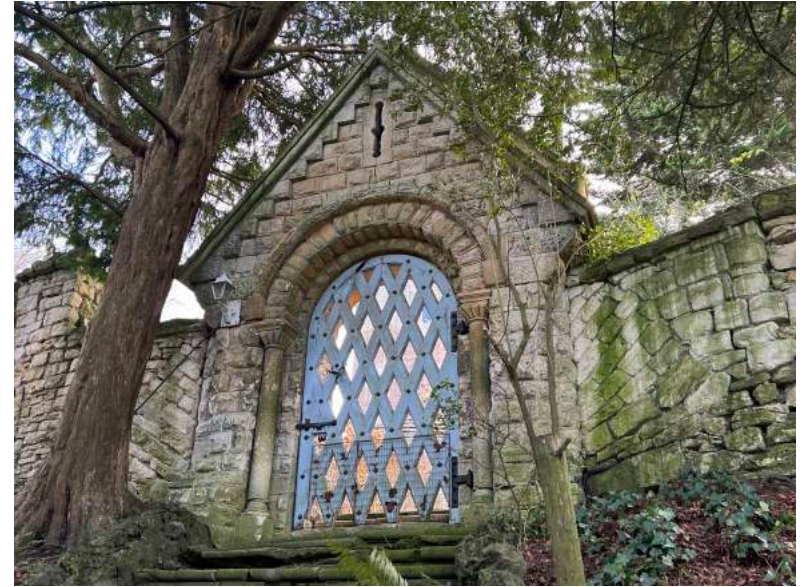
Figure 225 Northern gate, outside face.
