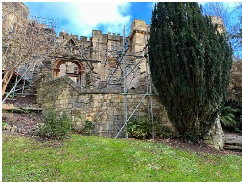
Figure 236 /stair up to Ladies' Gate , upper half.
