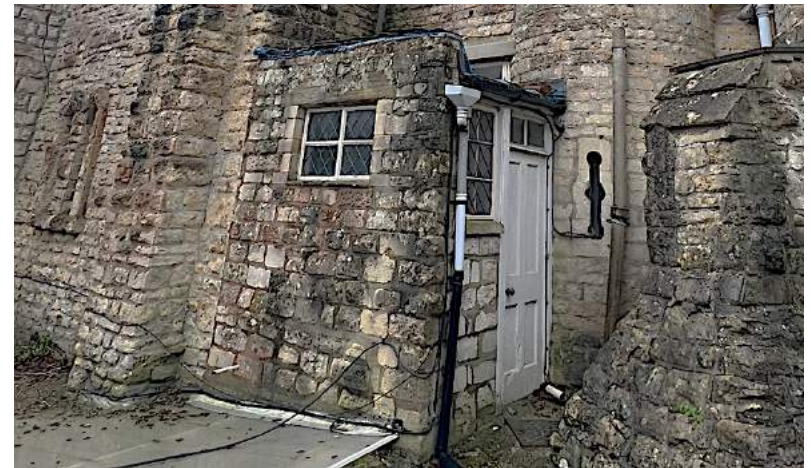
Figure 246 East elevation, modern bathroom extension.
