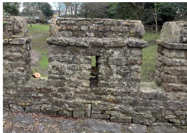
Figure 218 Bridge, north-east elevation, detail of merlon construction.
