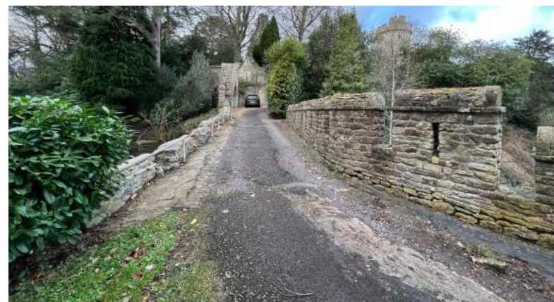
Figure 217 Bridge, view north over bridge, showing parapets; the wear in the middle of the drive, in the foreground, may possibly be the surviving top of the original north-east elevation.
