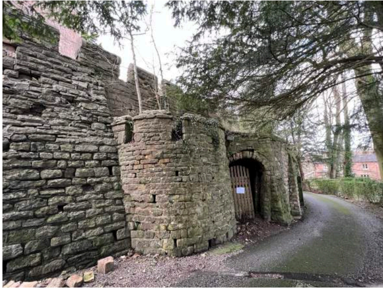
Figure 224 Boundary wall, to north-east of house.
