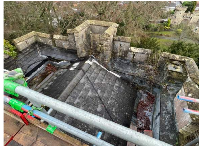
Figure 270 Eastern end of Drawing Room roof.
