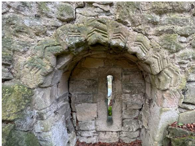
Figure 228 Seat, detail of salvaged Romanesque voussoirs with chevron moulding.
