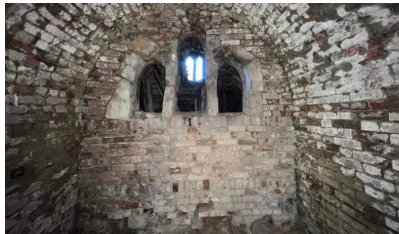
Figure 215 Within one of the vaults of the original bridge, showing the brick inner face of the original north-east elevation.
