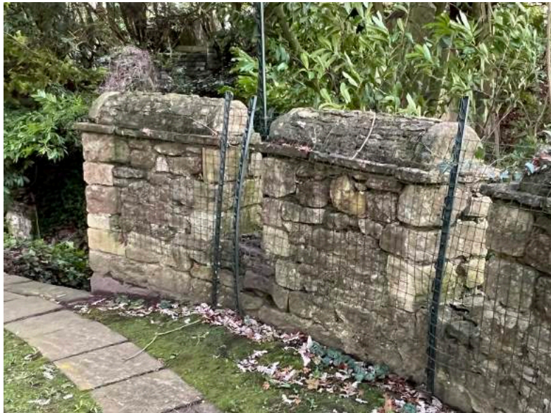
Figure 222 Boundary wall, typical merlon.
