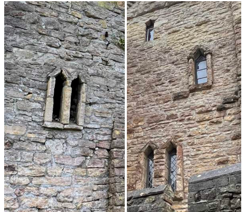
Figure 223 Windows of bridge (left) & north-east wing.
