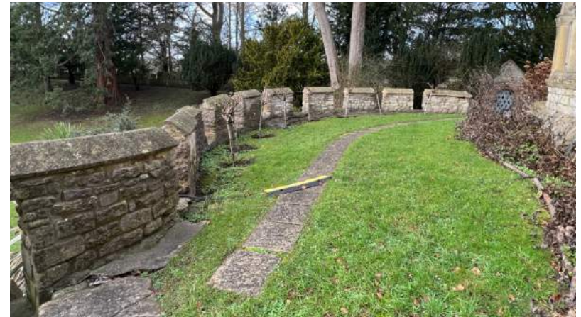
Figure 244 Terrace bastion around the Fernery .
