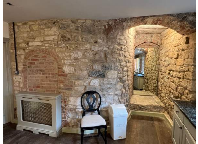
Figure 64 Kitchen, southern end.
