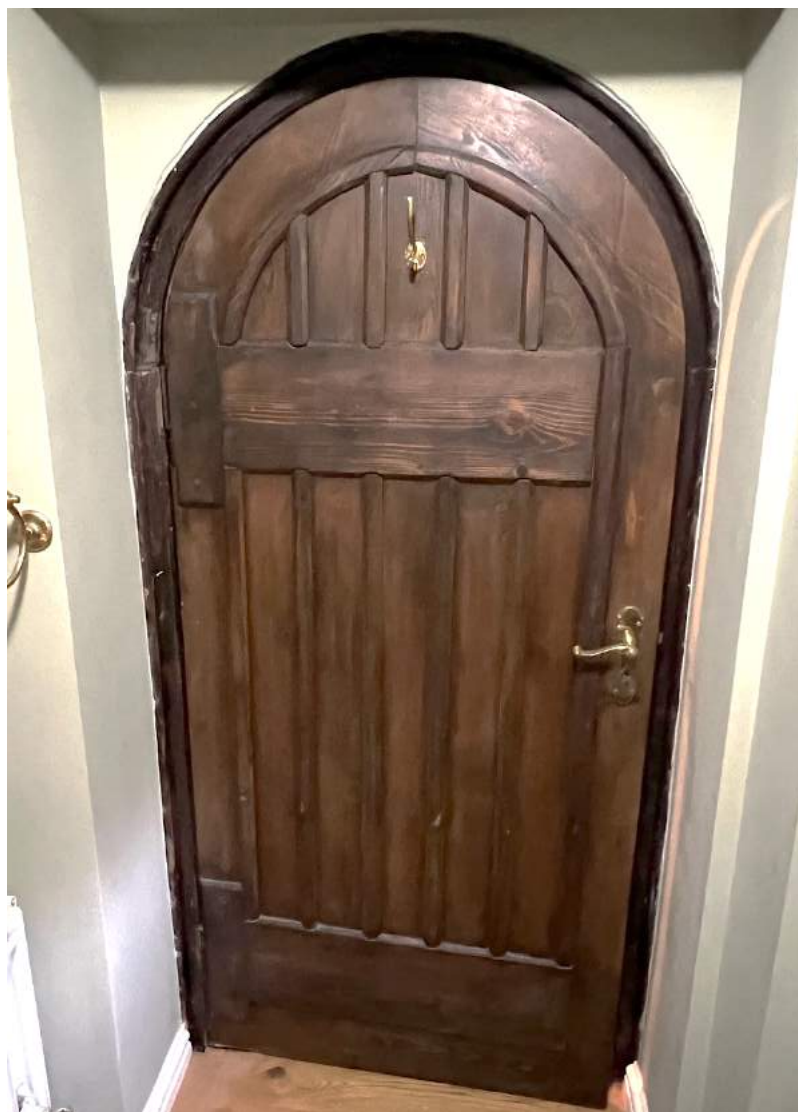
Figure 53 Door to cloakroom, inner face.
