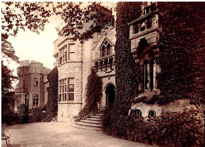
Figure 40 View north along the west front c.1914 (© Wiltshire Museum, Devizes; 2022.7013.2); the infill of the window to the right of the former arcaded balcony is legible as a patch of lighter, less weathered stone.
