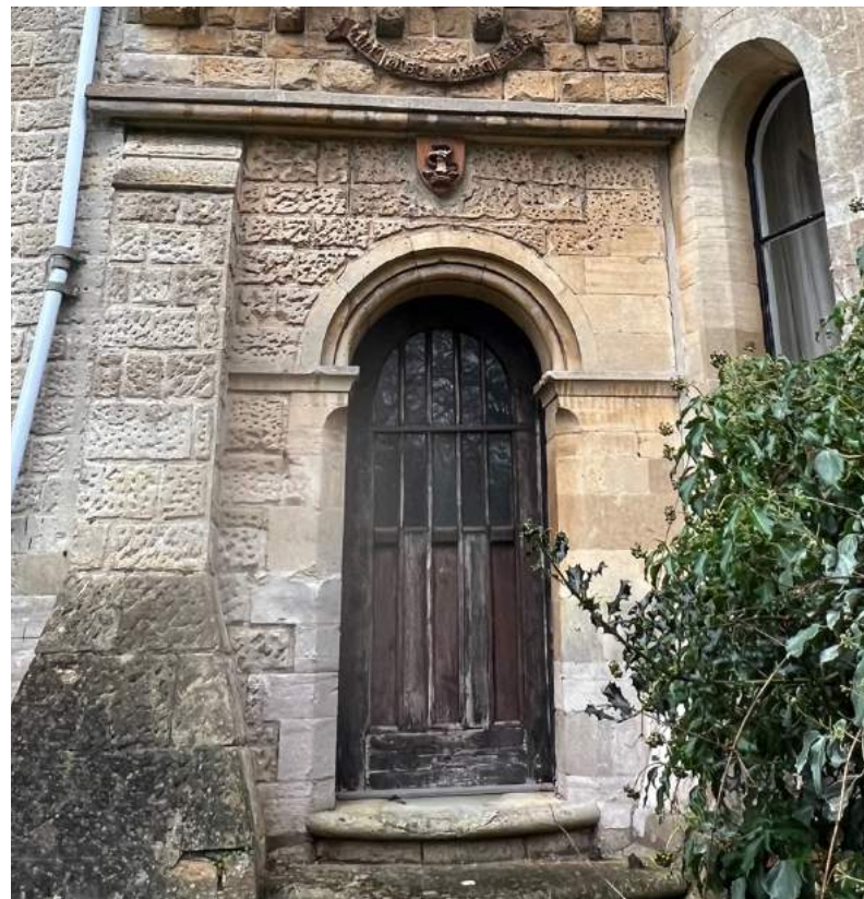
Figure 11 Garden porch, west front.
