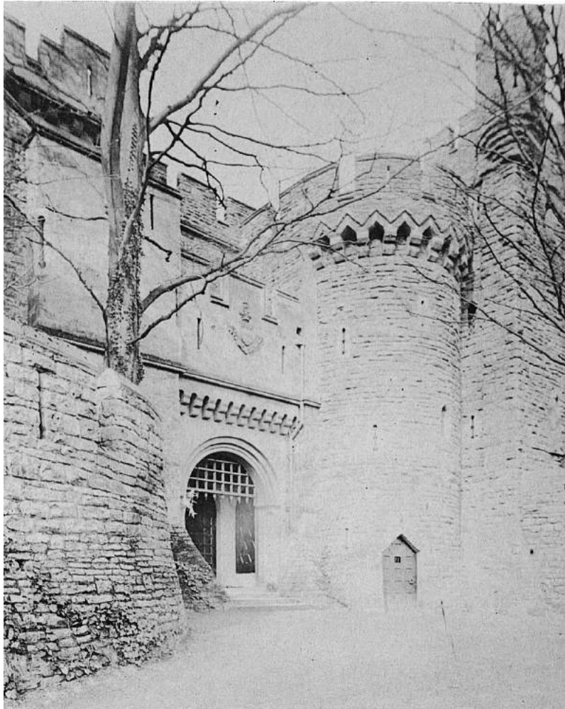
Figure 6 Photograph of the entrance from the south c.1883, showing Valentine Leach's earlier Portcullis Gate embedded in later rock-cut masonry (© Wiltshire Museum, Devizes; DZ/WJ:1983.7725).
