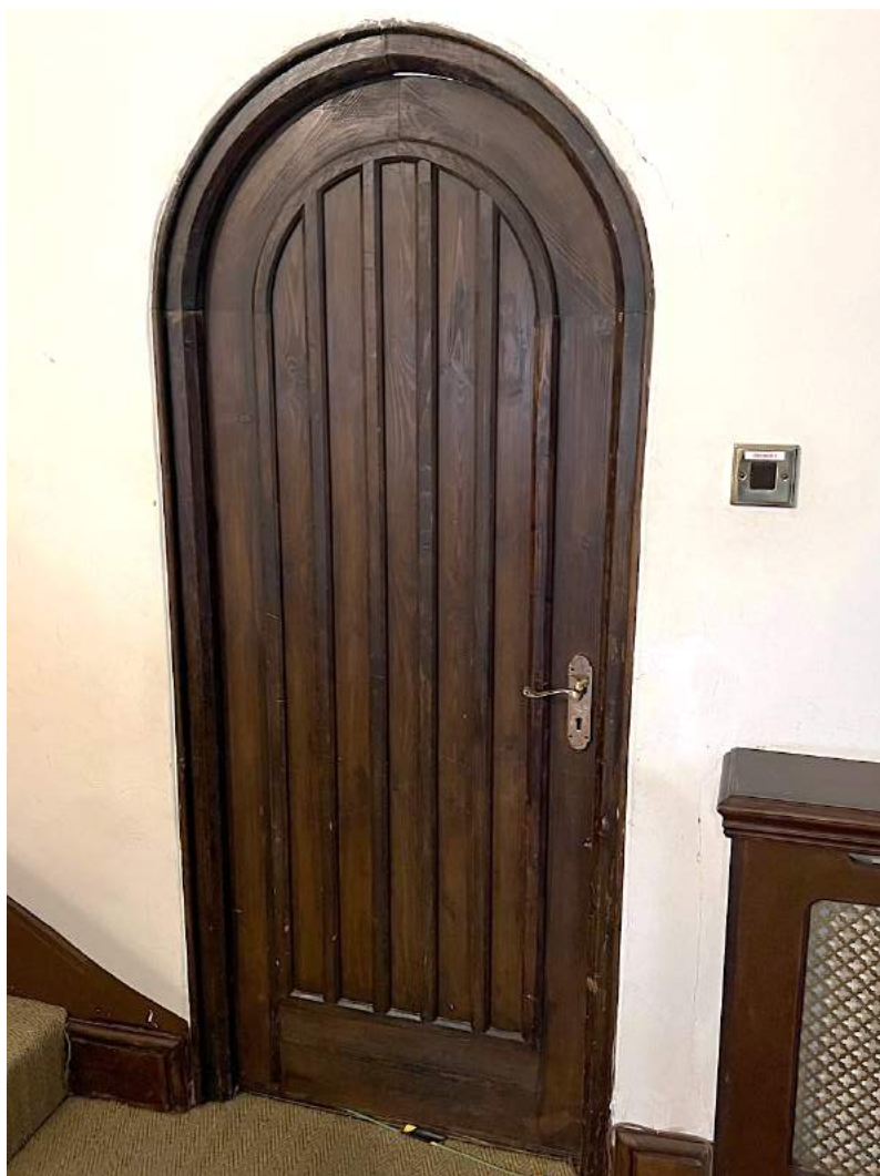
Figure 68 Kitchen, door from inner hall (hall face).
