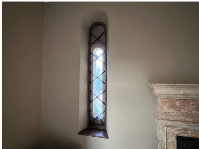
Figure 15 Probably original casement in first floor of dining room block.
