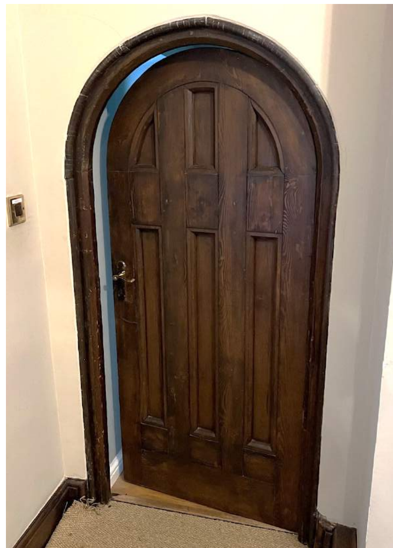
Figure 52 Door to cloakroom; outer face.
