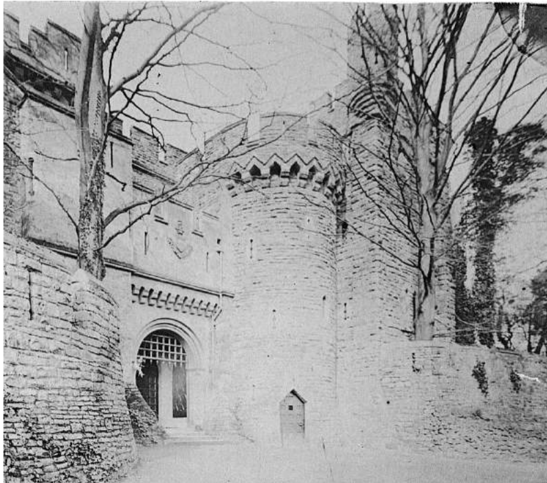
Figure 27 Photograph of the entrance from the south c.1883, showing Valentine Leach's ashlar entrance embedded in later rock-cut masonry (© Wiltshire Museum, Devizes; DZ/WJ:1983.7725).
