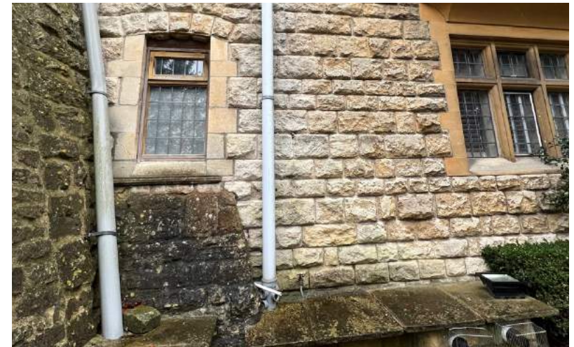
Figure 56 Exterior of cloakroom window.
