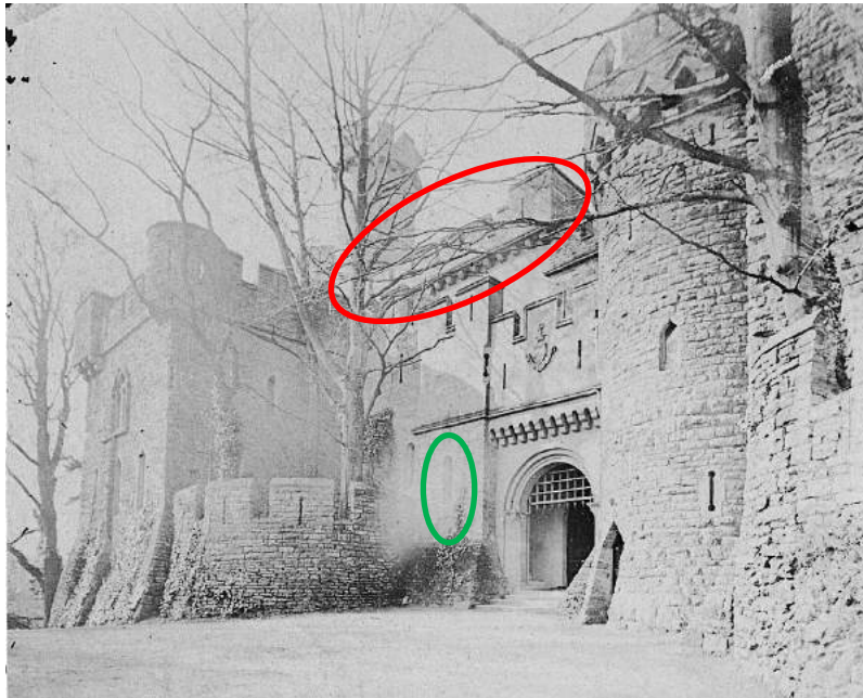
Figure 8 View of the entrance from the north, from the 1883 sales particulars (© Wiltshire Museum, Devizes; DZ/WJ:1983.7725), window visible in the 1843 sales particulars, eastern parapet of dining room block.
