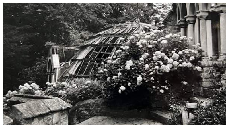
Figure 31 Conservatory & fernery from the south, photographed in March 1989 (Historic England Archive, BF077986 (89/519)).
