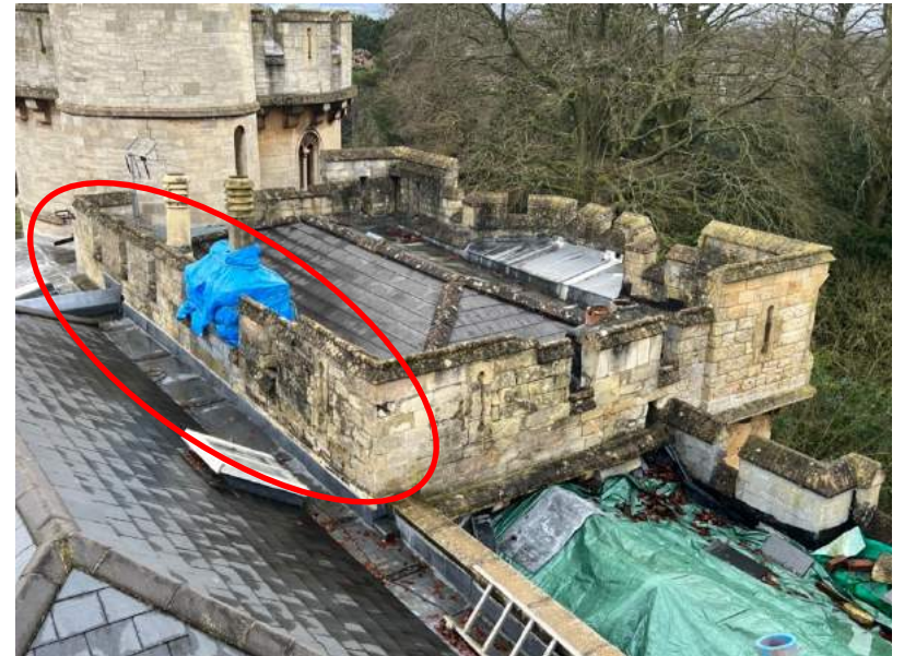
Figure 9 Eastern parapet of dining room block.
