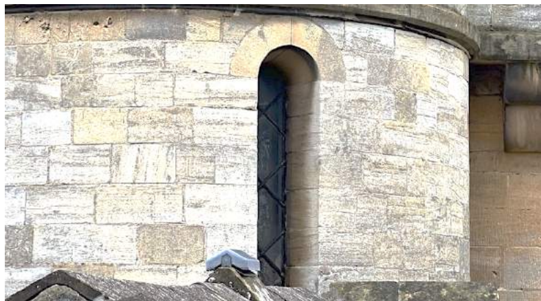
Figure 14 South tower turret, window overlooking roof of dining room block, with probably original casement.
