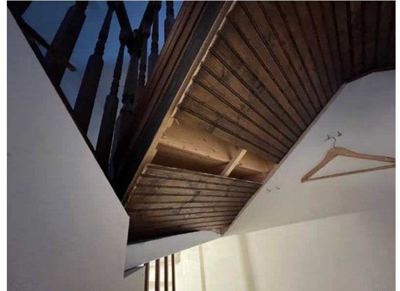
Figure 59 Back stair, soffit showing modern construction.
