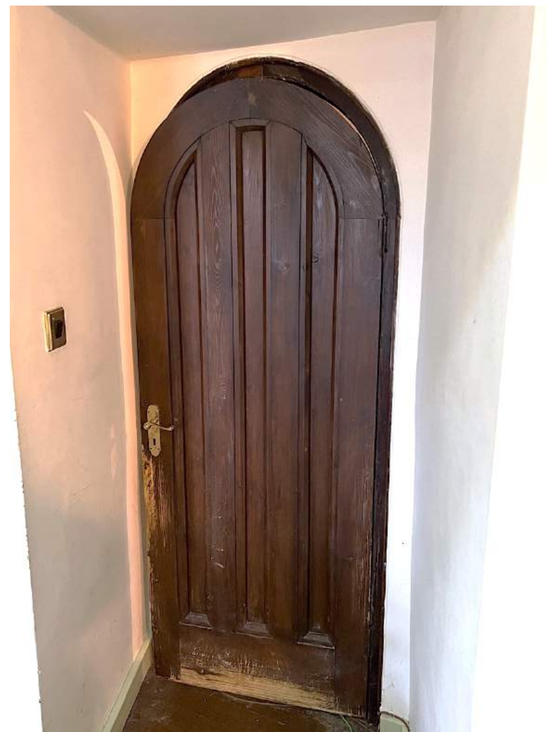
Figure 67 Kitchen, door from inner hall (kitchen face).
