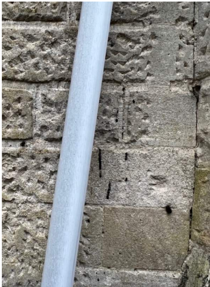
Figure 10 West front of dining room block, masonry to right of bay window.
