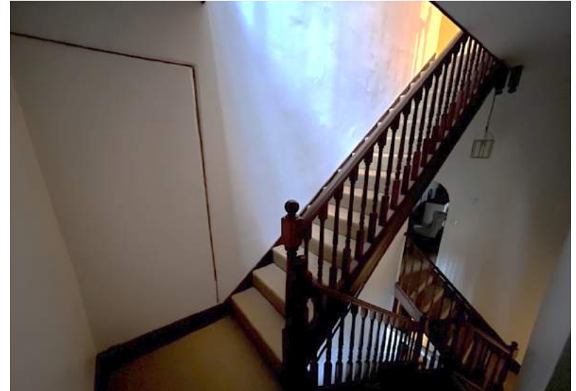
Figure 61 Back stair, half-landing showing blocked door to adjacent wing.
