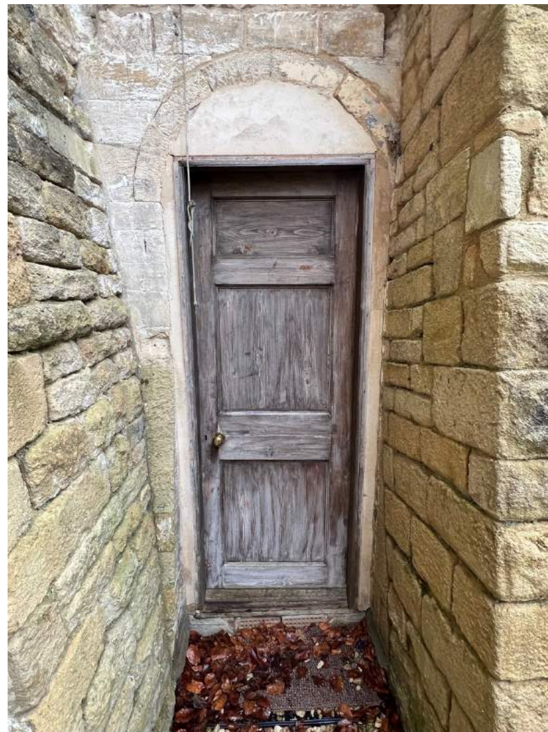
Figure 66 Garden door from kitchen, external face.
