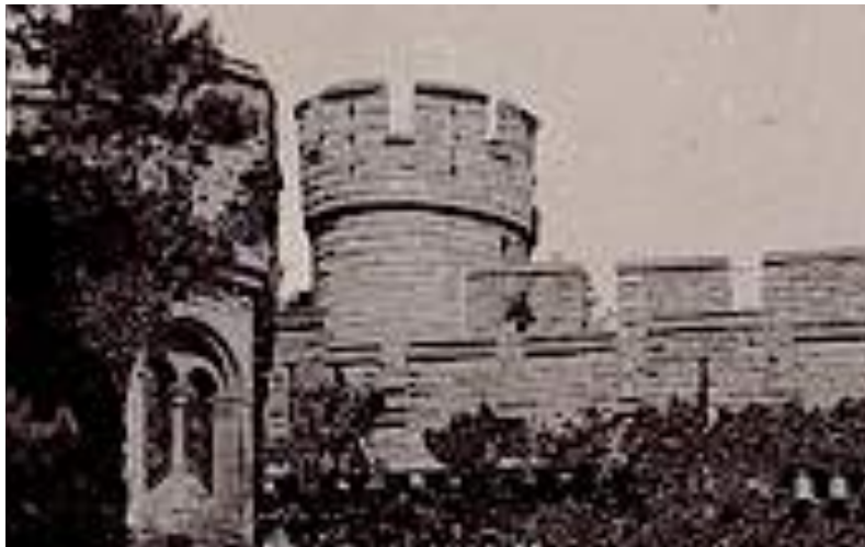
Figure 19 Detail of abutment of turret to parapet of wing to east of gallery in 1888 (© Wiltshire Museum, Devizes; 2022.7013.10).
