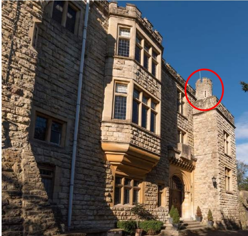
Figure 38 East front from the south, contemporary view showing Rich extension; the same round turret is encircled on both for reference.
