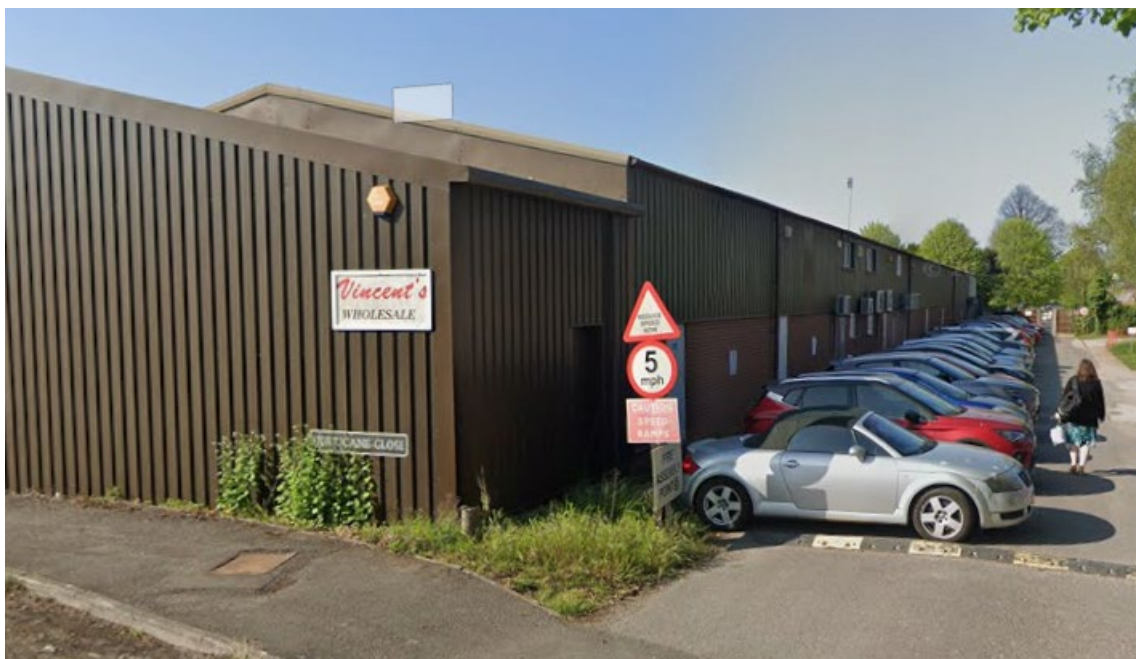
Figure 6 - Plant on rear elevations of commercial units on Hurricane Close (directly adjoining the application site)
