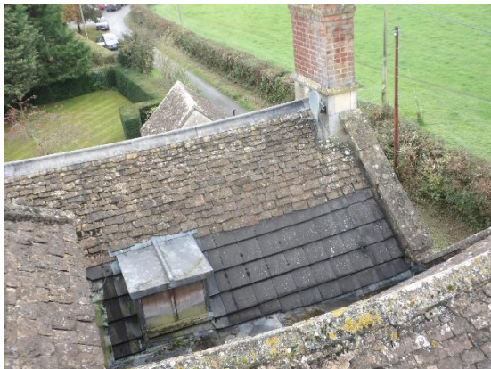
(North west roadside gables elevation roof coverings with a mixture of old stone and replacement concrete tiled covering and boarded up dormer window)
