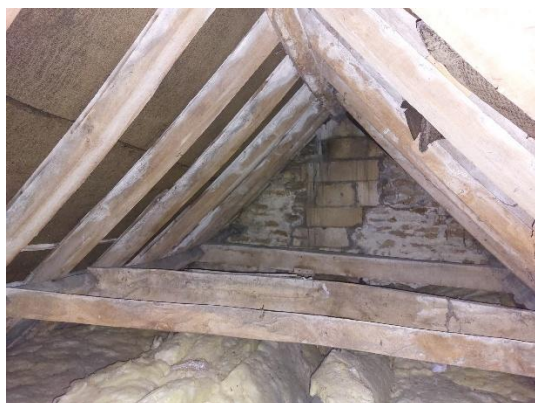
(Roof void from bedroom, with older style and deteriorating 1F bitumen felt, some timber decay noted from water penetration)
