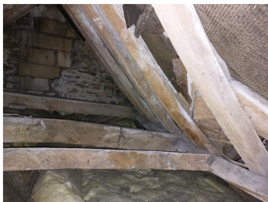
(Roof void from bedroom, with older style and deteriorating 1F bitumen felt, some timber decay noted from water penetration)
