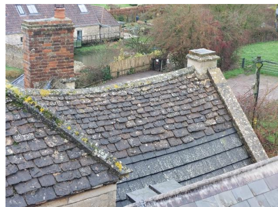
(North west roadside gables elevation roof coverings with a mixture of old stone and replacement concrete tiled covering and boarded up dormer window)
