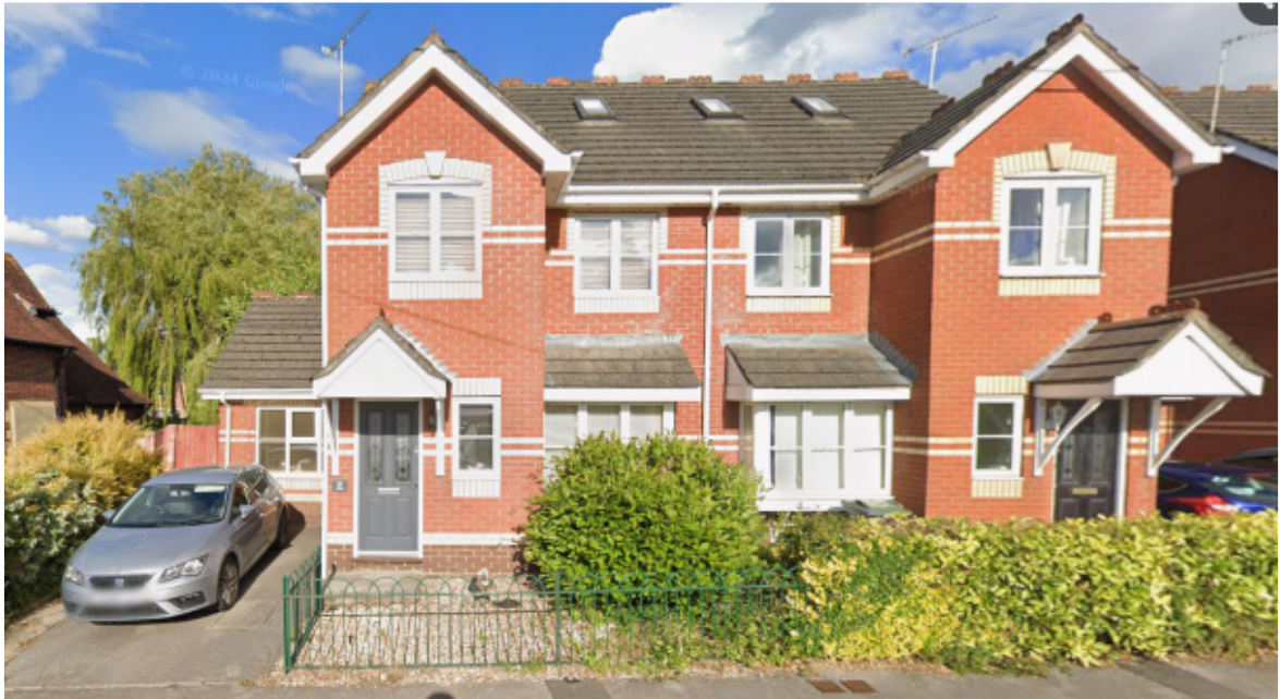
Existing residential housing adjoining southern boundary site – Semi-detached with off street parking
