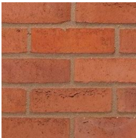
Red facing brickwork
