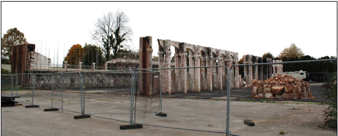
Photo 14. Remains of recently burnt-out Grade II* listed double Hangar 3
