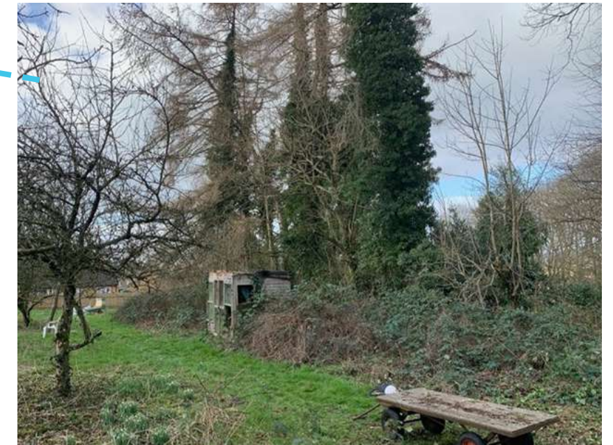
Summer house in disrepair, with unmanaged vegetation. Demonstrates extent of previous curtilage.
