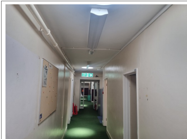
Photograph 7. Internal view along the central corridor.
