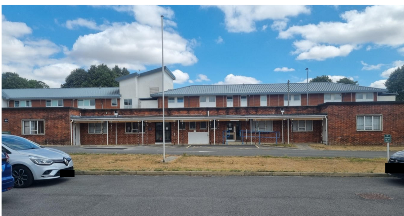
Photograph 1. General view in the foreground of the front southwestern elevation of the building.
