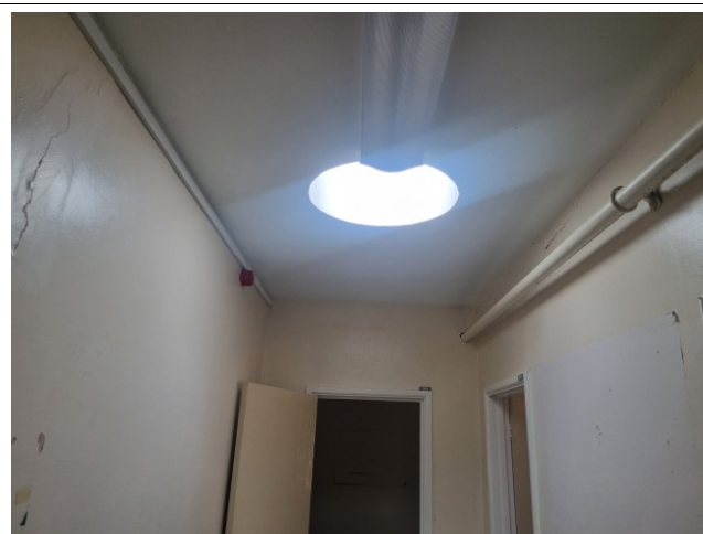
Photograph 8. Light from the roof skylight in the corridor.
