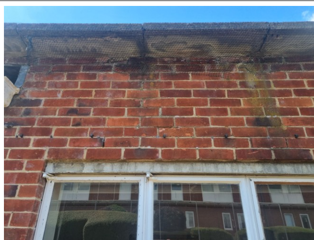
Photograph 9. Preventative netting installed under the eaves.
