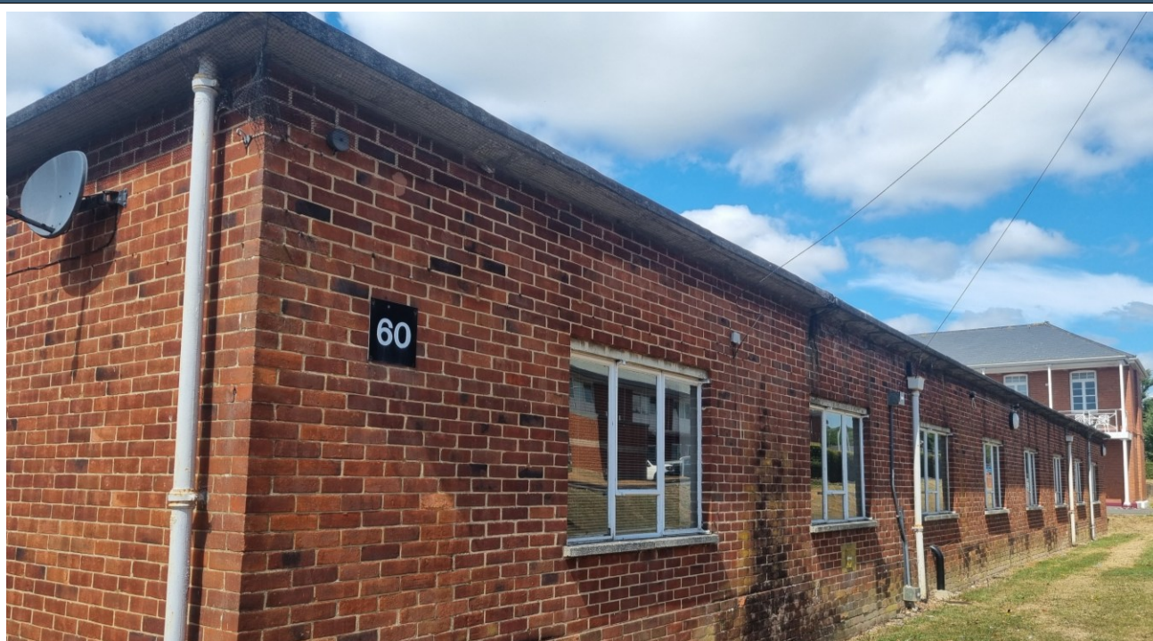
Photograph 2. View along the rear of the building alongside Kirkee Road, looking southeast towards the main gate.
