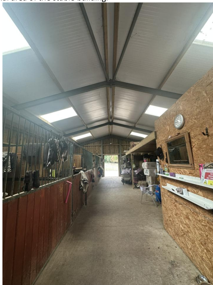
Photograph 8: Internal area of the stable building.
