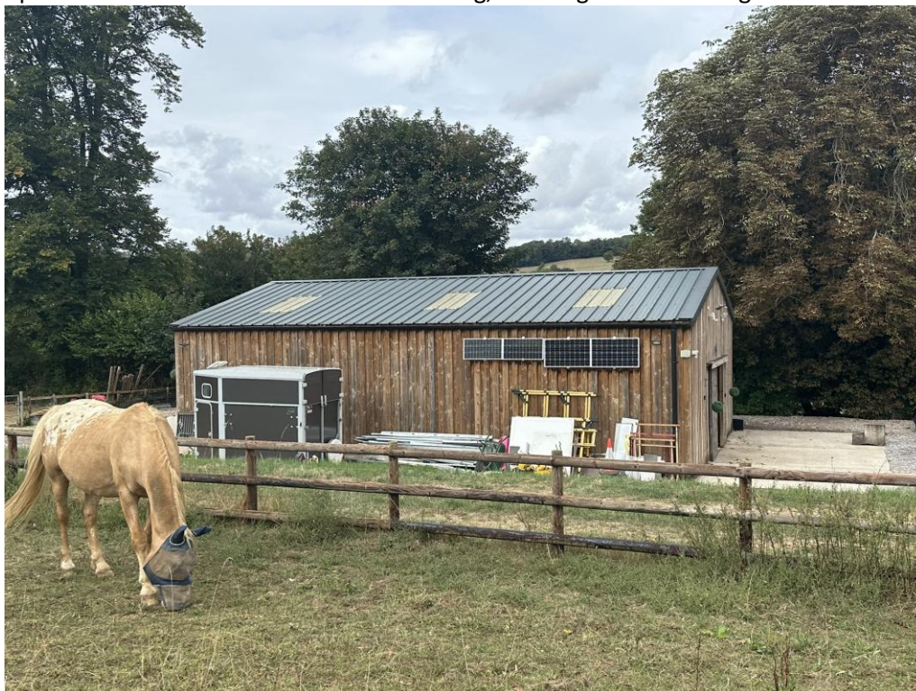
Photograph 9: South elevation of the stable building, showing the modified grassland to the south.
