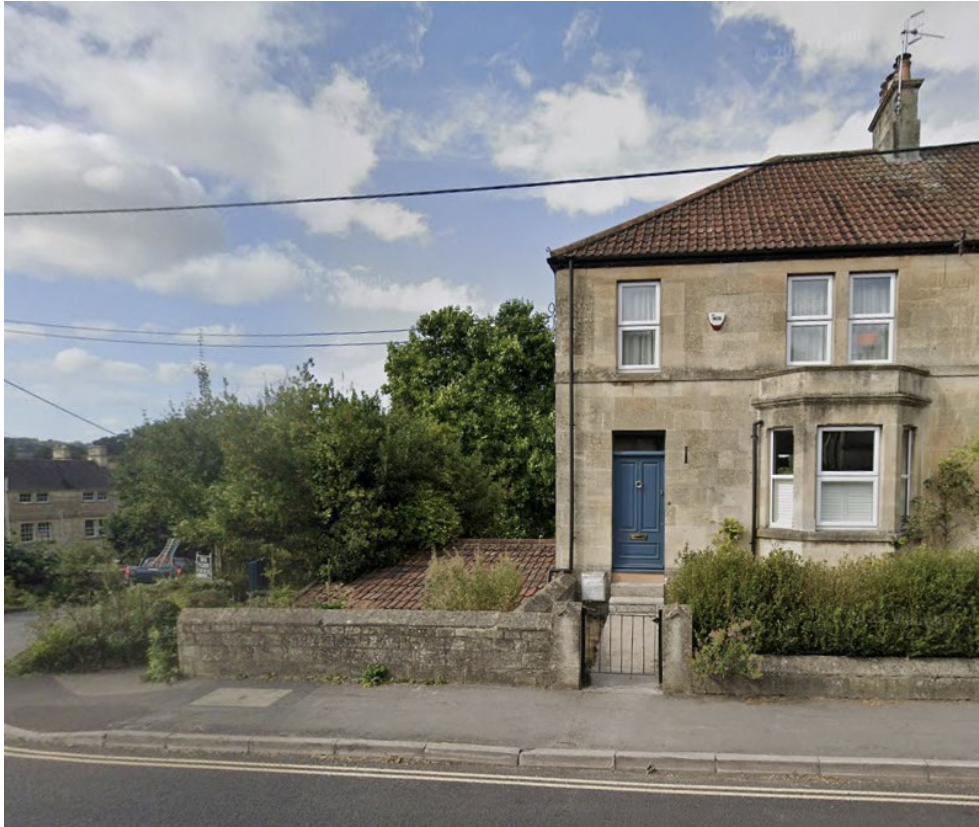
Existing Front street view
