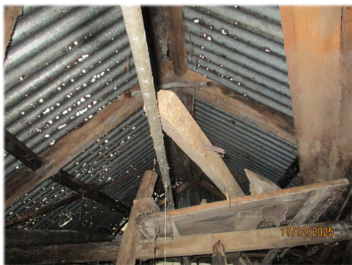
Shed 1 interior with degraded roof (left) and established webbing (right)
