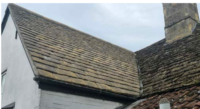
No. 40 Shurnhold - Adjoining Roof/Tiles
