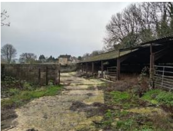
Photograph 5. Hardstanding yard area and building B1
