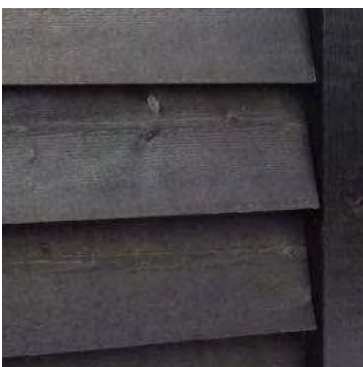
Dark stained horizontal weatherboard cladding
