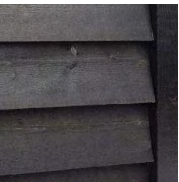
Dark stained horizontal weatherboard cladding
