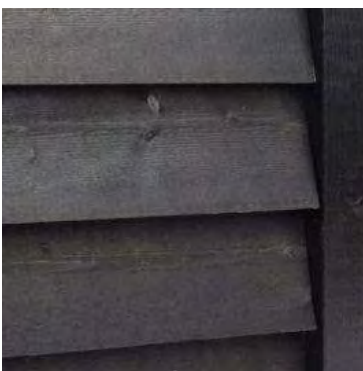
Dark stained horizontal weatherboard cladding
