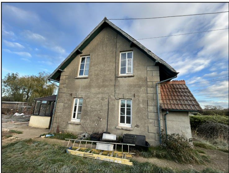
PHOTOGRAPH 2 EXISTING SOUTH ELEVATION
