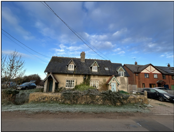
PHOTOGRAPH 1 EXISTING EAST ELEVATION
