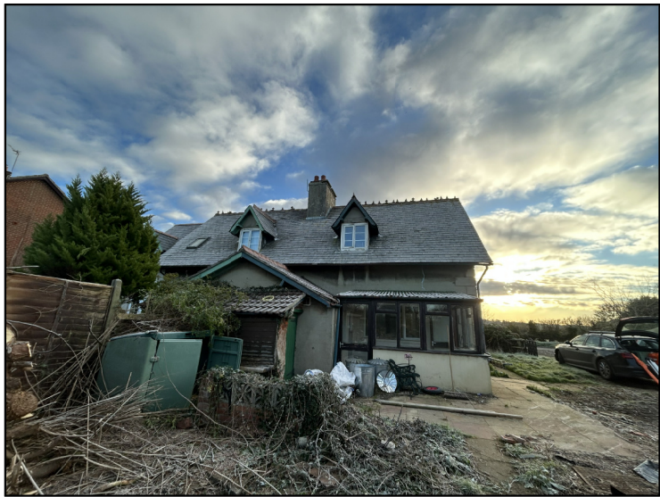
PHOTOGRAPH 3 EXISTING WEST ELEVATION
