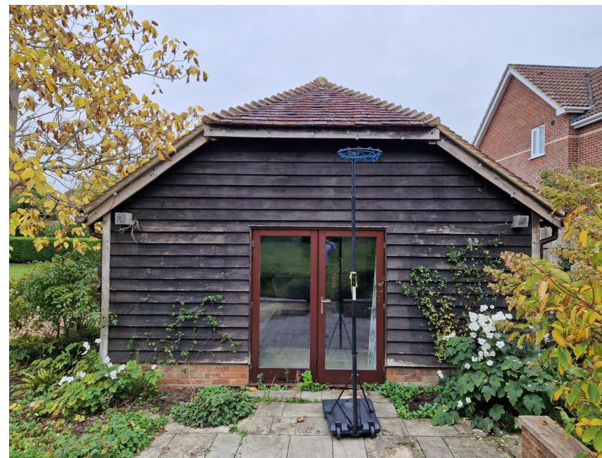
Existing garden room
