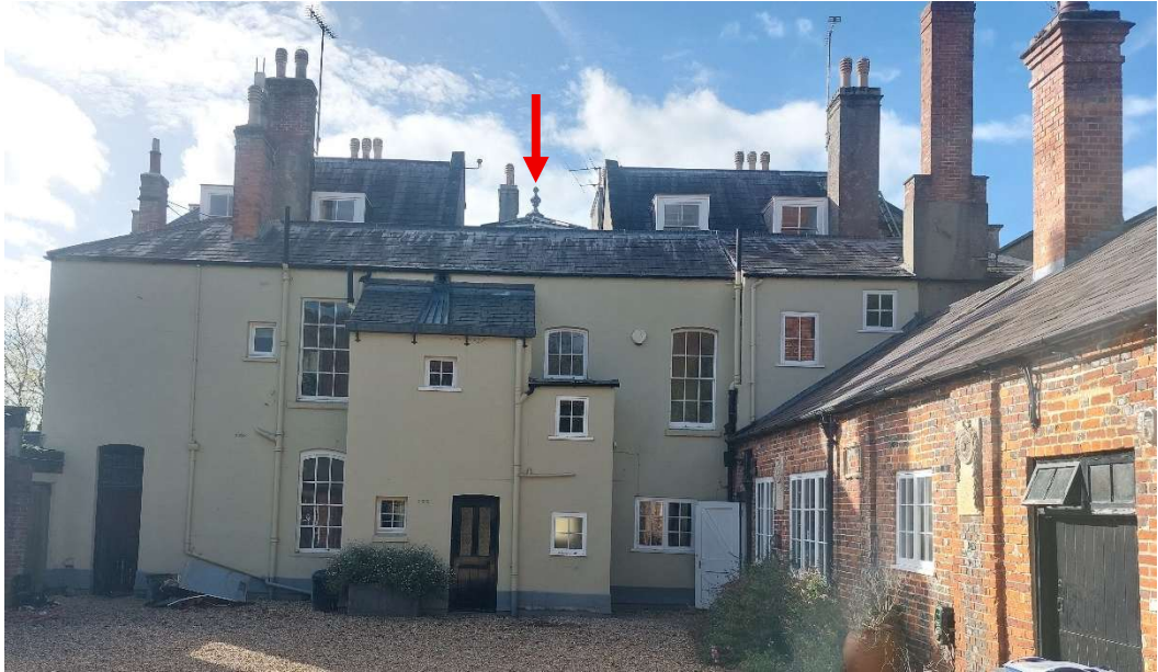
Figure 2 The rear elevation of Rainscombe House. The finial of the lantern can just be seen above the ridge of the rear range (arrowed).
