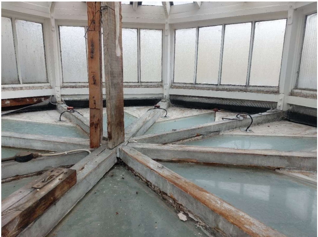
Figure 5 Interior of the lantern showing the timbers to the glazing at the base of the lantern.
