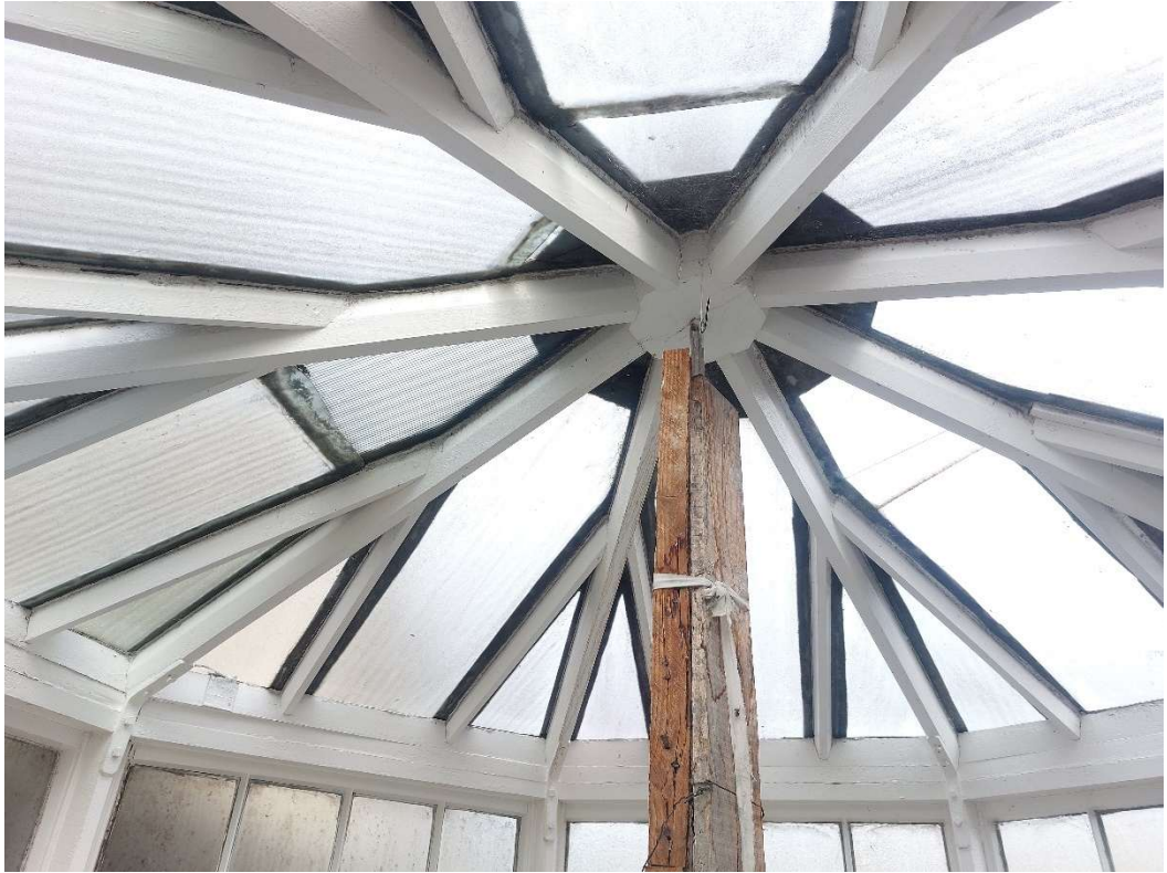
Figure 6 The interior of the lantern showing the underside of the roof structure.
