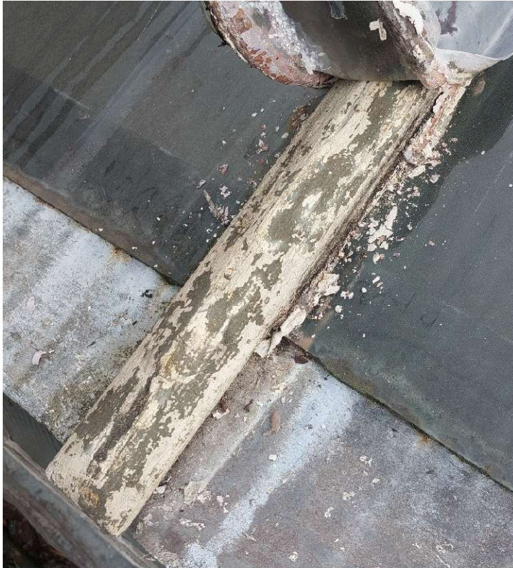
Figure 4 Exposure of one of the ribs to the roof of the lantern.
