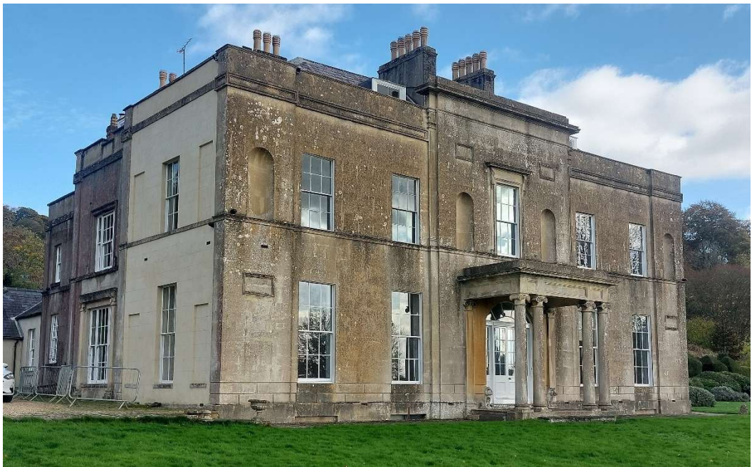
Figure 1 The front elevation of Rainscombe House
