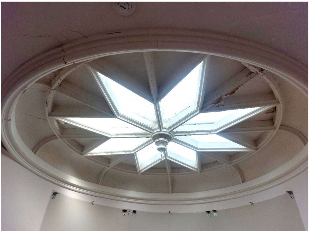
Figure 3 The lantern above the principal stair.
