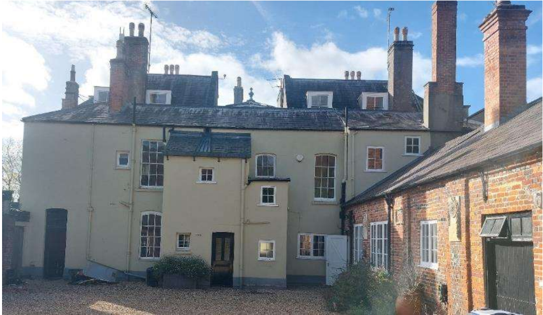
Figure 2 The rear elevation of Rainscombe House.
