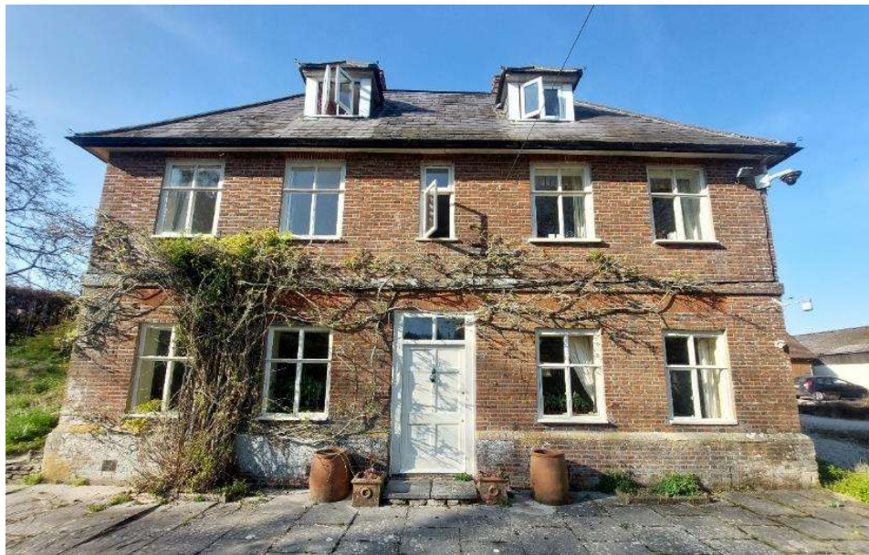
Figure 4 Front, south elevation.
