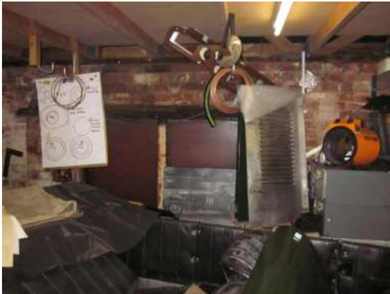
Historic west wall
