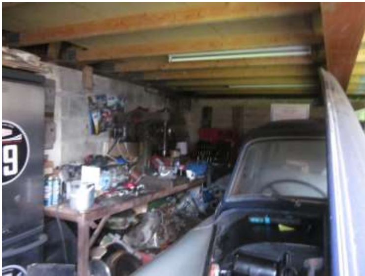
'Modern' blockwork walls and trussed rafters
