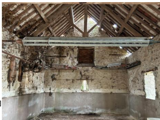
Figure 10: Internal photo of barn 4, showing trusses
