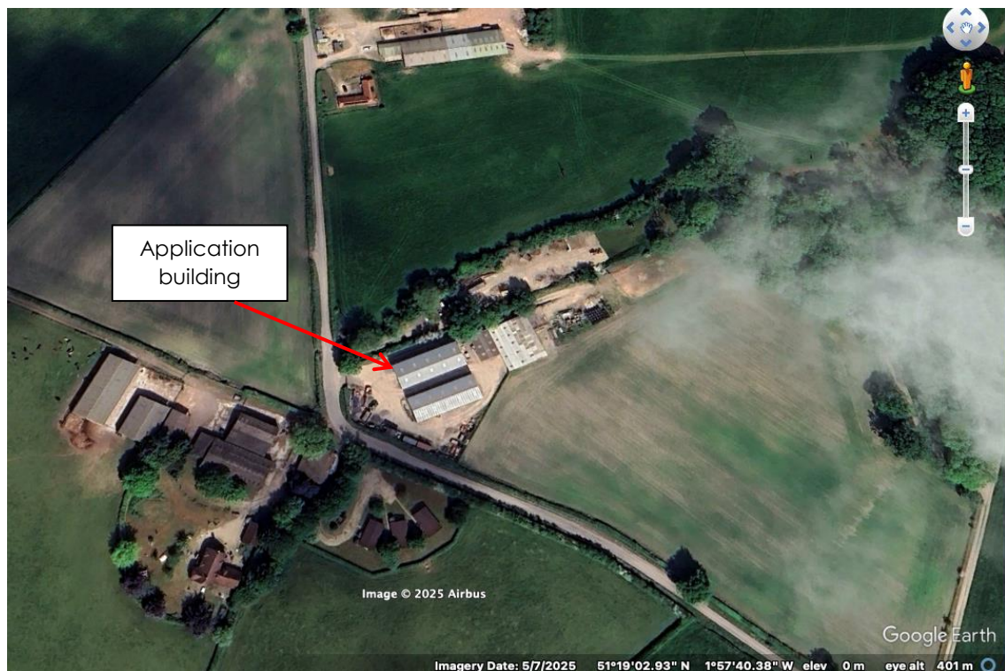
Figure 2 – Application building within the farmyard
