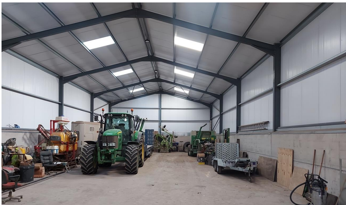
Figure 4 –internal view of application building
