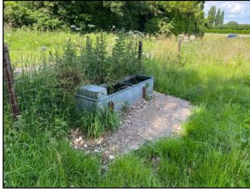
Figure 3 – hardstanding beneath the water trough.
