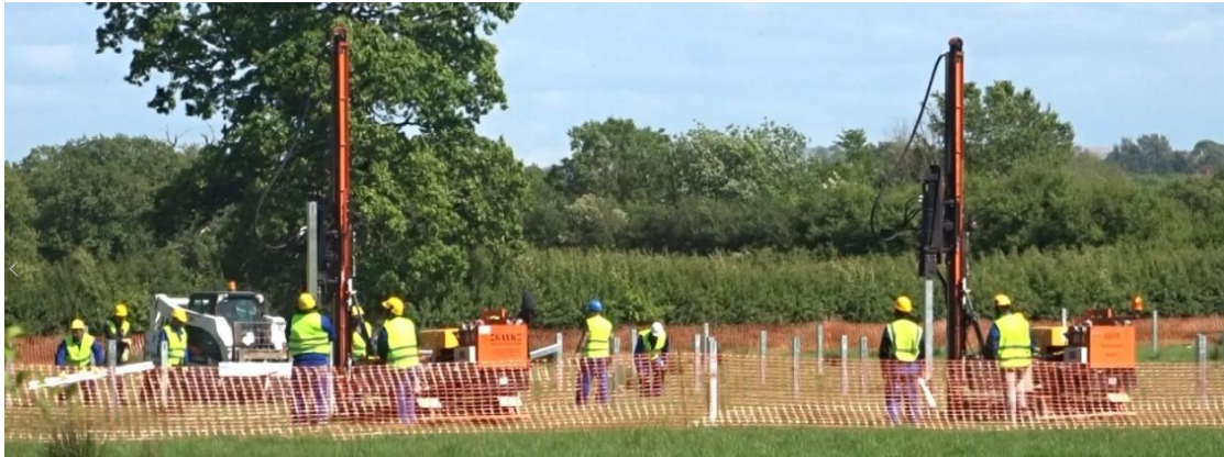
Photo 2: Posts Being Installed
