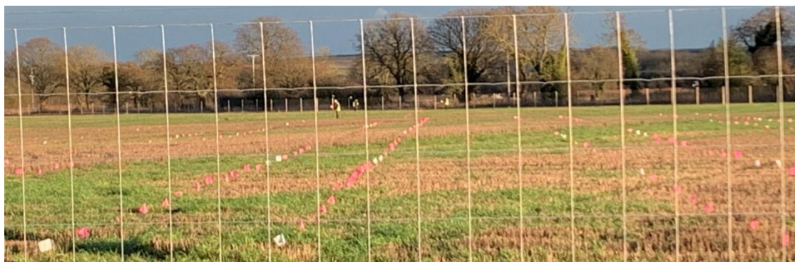
Photo 1: Marking Out in Progress
